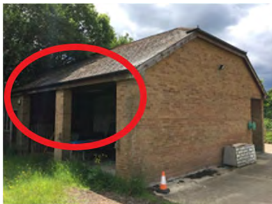
Photo 93 Building B3 – BLE emergence point
