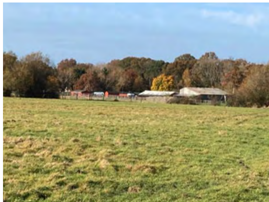
Photo 91 Buildings B13 – B17
