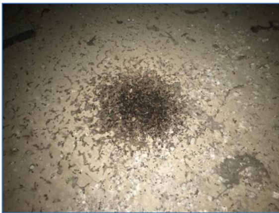
Photo 53 Cluster of bat droppings pile 1 (B3)
