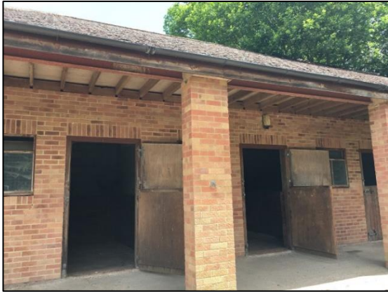
Photo 45 Barn structure (B3)
