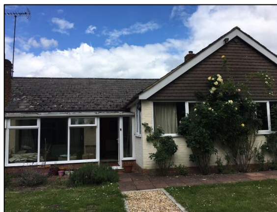
Photo 34 Residential dwelling (B1)
