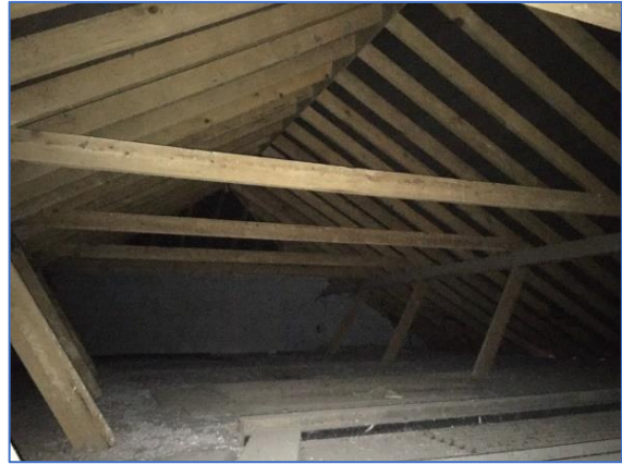
Photo 52 Barn loft void (B3)
