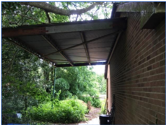
Photo 47 Barn structure (B3)
