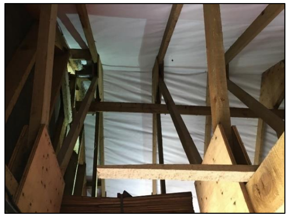
Photo 44 Internals of outbuilding (B2)
