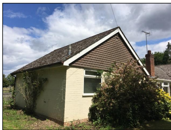
Photo 36 Residential dwelling (B1)
