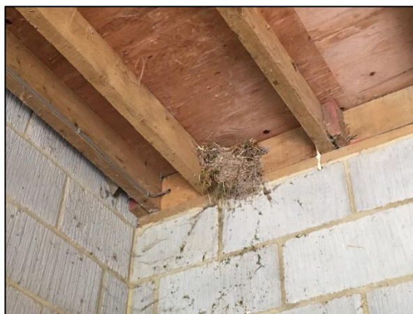
Photo 67 One of ten house martin nests within B3
