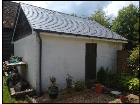
Photo 40 Brick outbuilding (B2)
