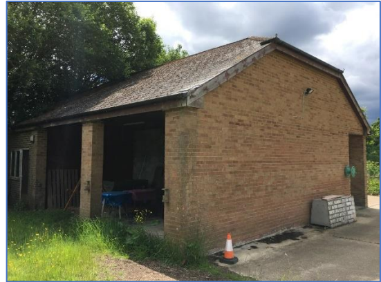
Photo 46 Barn structure (B3)
