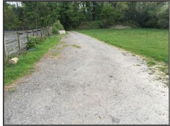
Photo 31 Compressed concrete path
