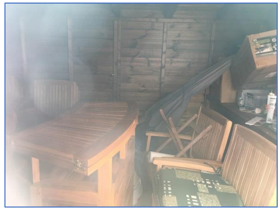
Photo 62 Timber shed internals (B6)
