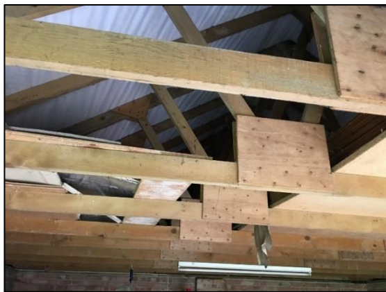
Photo 43 Internals of outbuilding (B2)
