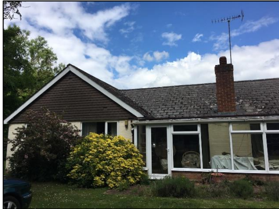
Photo 39 Residential dwelling (B1)
