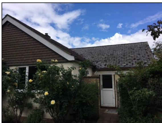
Photo 33 Residential dwelling (B1)
