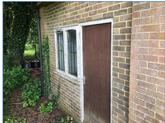
Photo 48 Barn structure (B3)
