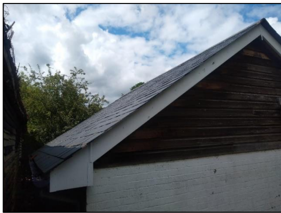
Photo 41 Brick outbuilding (B2)
