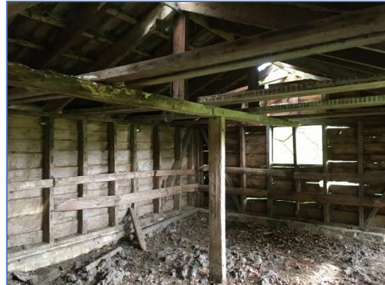
Photo 64 Timber outbuilding internals (B7)
