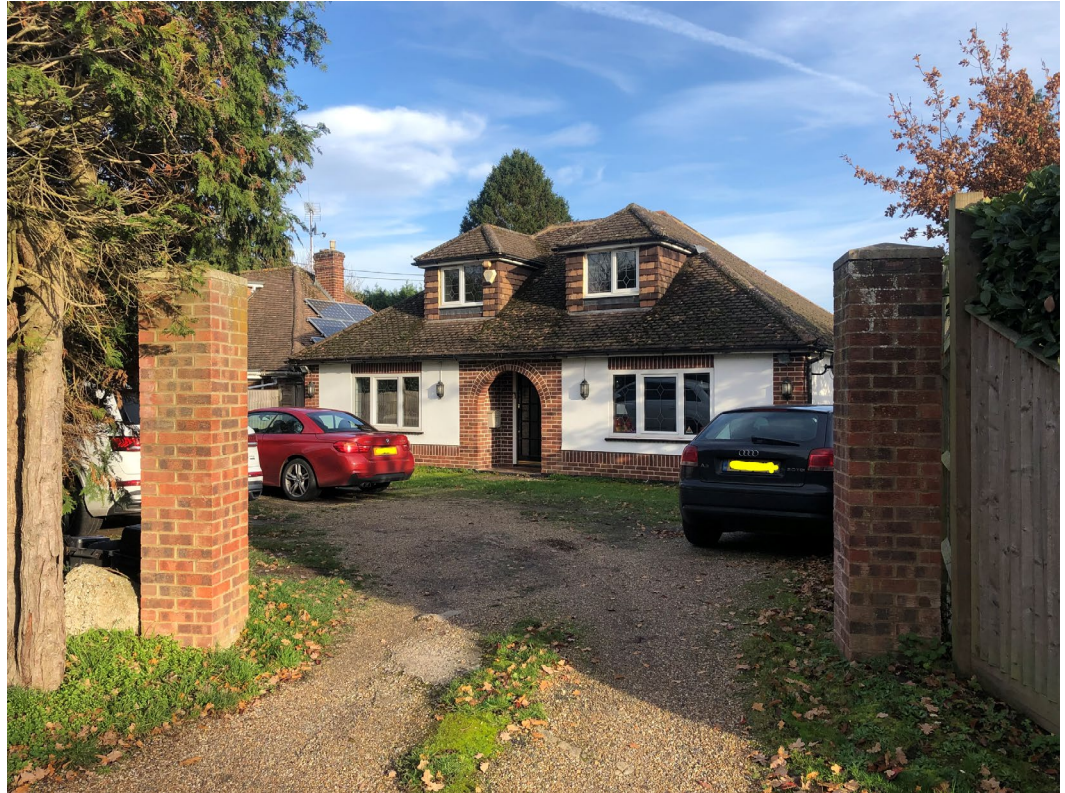
Figure 1 : View of site from Entrance @ Grovelands Road
