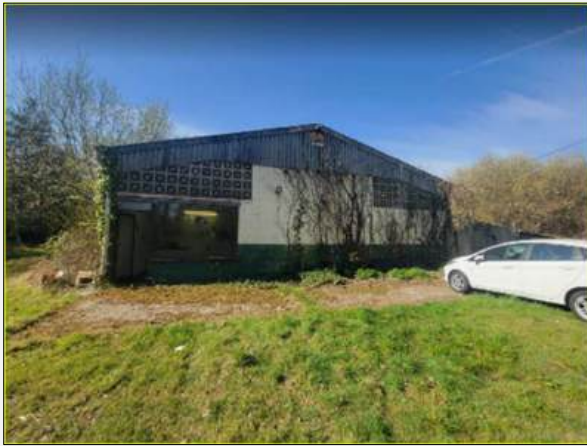
Plate 5: large barn which forms part of a wider barn complex. The roof is comprised of corrugated metal, and walls are comprised of both cement brick and corrugated metal
