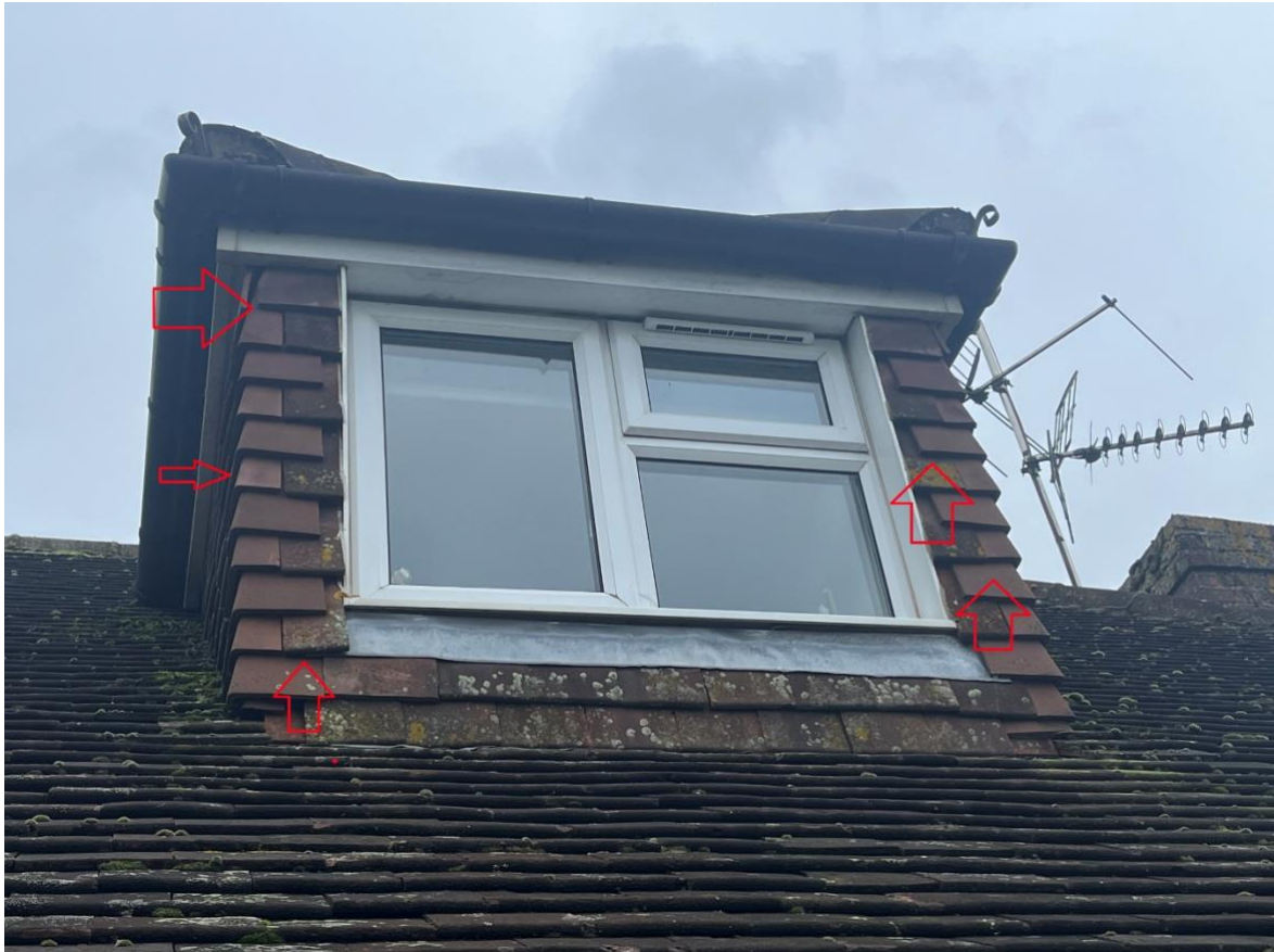
Figure 4. Wet dormer looking east: Red arrows indicate potential openings for crevice roosting bats.
