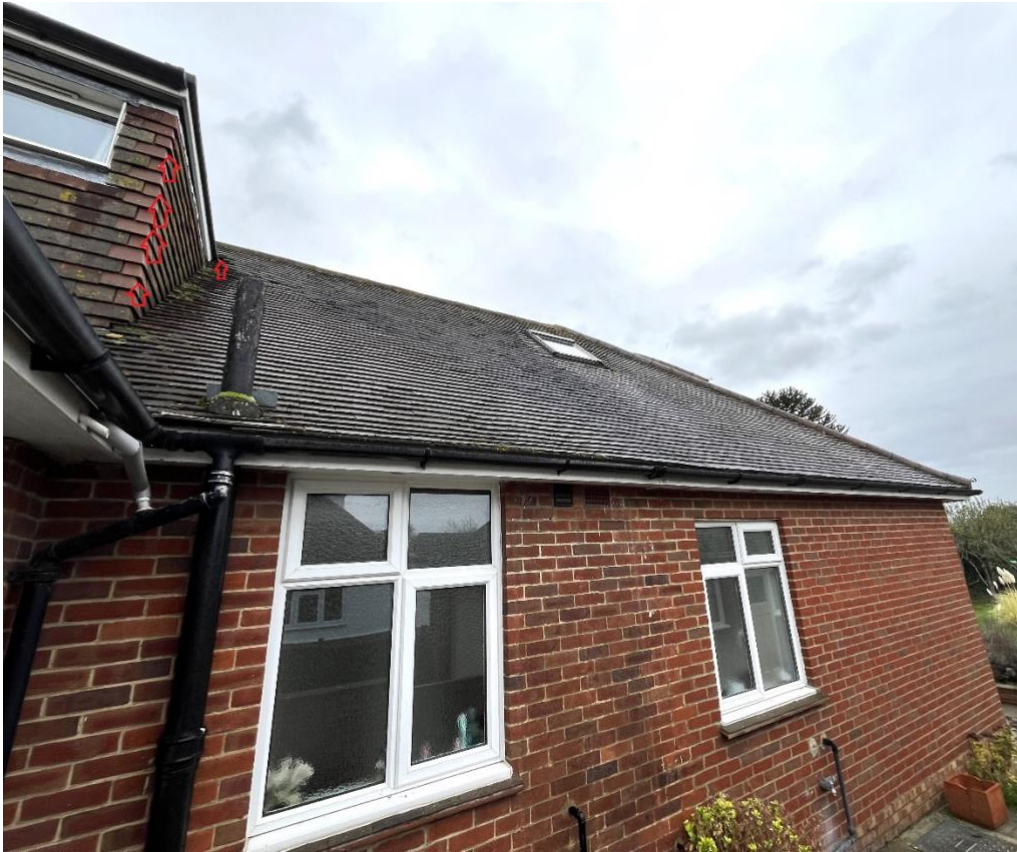
Figure 6. South face of rear extension looking northeast. Red arrows indicate potential openings for crevice roosting bats.
