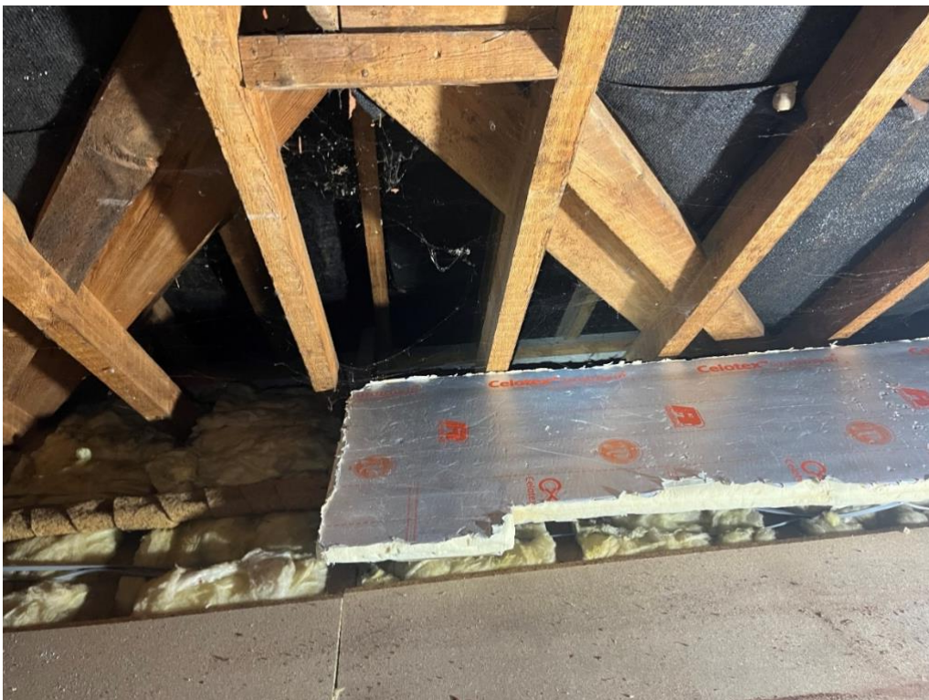
Figure 6. Loft looking west.
