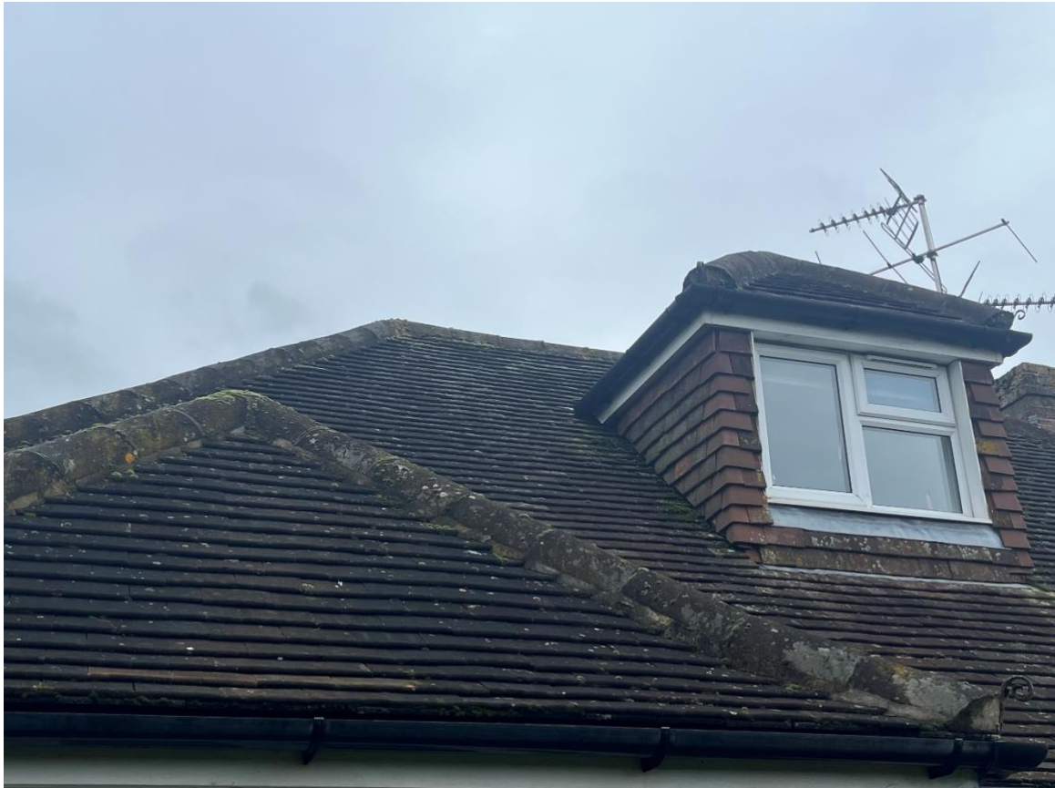
Figure 2. Western elevations northern half looking southeast.
