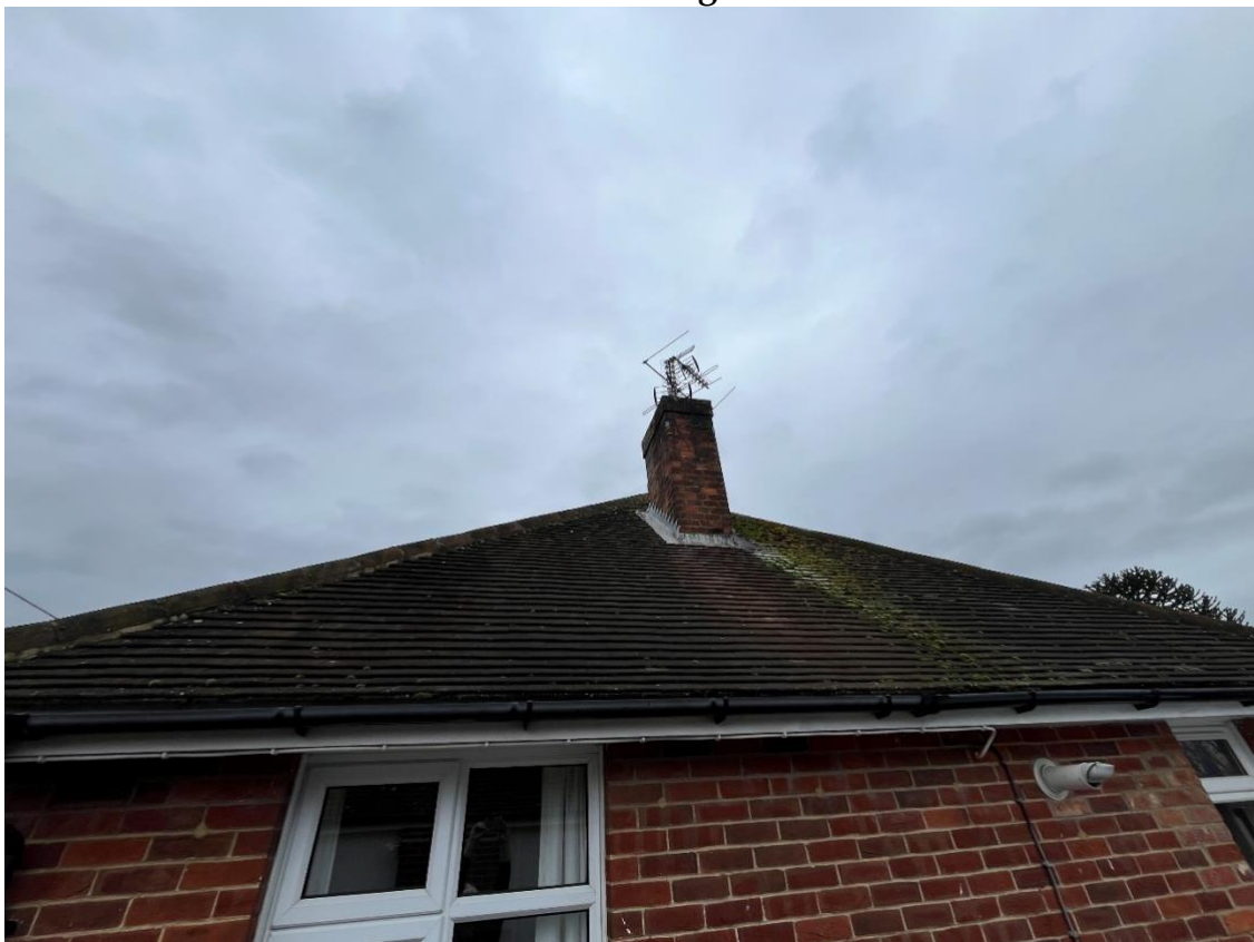
Figure 5. South hip looking north.
