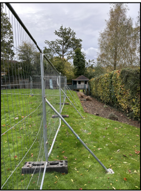
Protective Barrier (P.B.) (S.T.P.) A support bar will be placed at a 45-degree angle at each end of the Heras panel and pinned to the ground using a soil pin.
