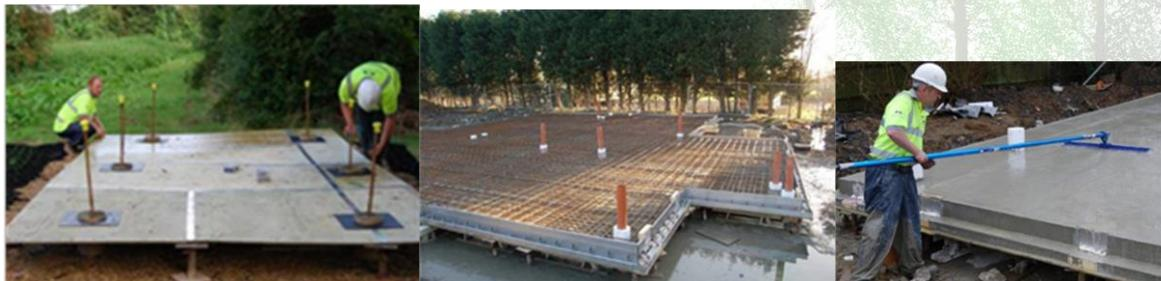
The completed deck with pile overlays made of flexible material prevents concrete from the slab pour leaching onto the ground surface. Similarly, the aluminium strips between the sheets of ply prevent concrete reaching the ground surface.
