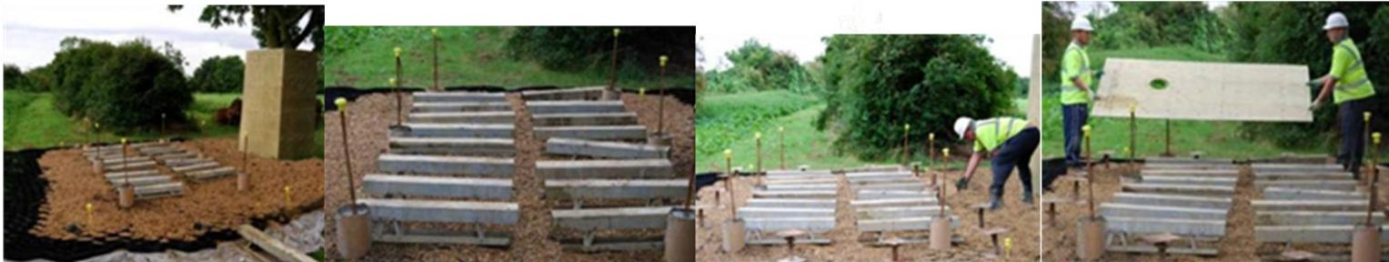
Perimeter jacks are laid around the edge of the footprint to allow fine level adjustments to be made.
