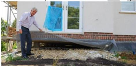
This picture shows the finished voided system. The piles supporting the slab can be seen as well as the clear void the Housedeck system leaves. The pea shingle and CellWeb under the slab are also visible and the geotextile membrane which prevents materials entering the void can be seen attached to the underside of the slab.
