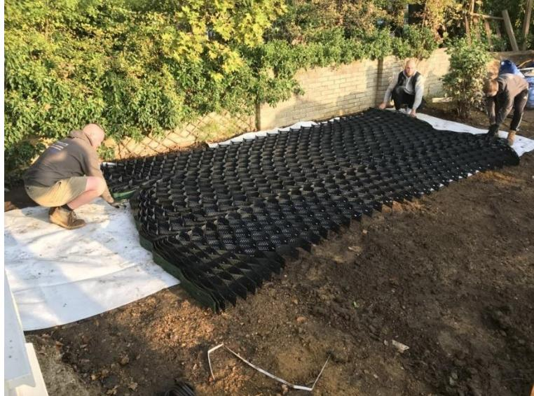
Pin the edges of the cellular confinement with wooden or metal pins and add wooden retention board.
