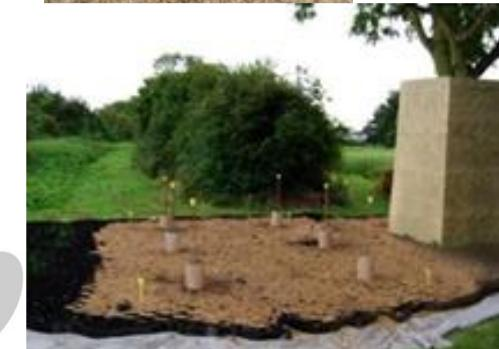
Each pile position is sleeved using a polythene coated cardboard tube to prevent concrete from the pile leaching into the root zone.
