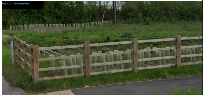
Image 1: May 2023, showing where the headwall guardrails are clearly visible.
