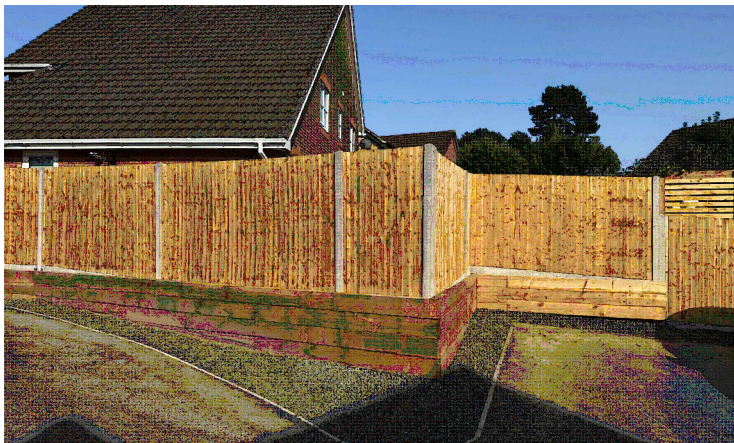
View from road facing East
