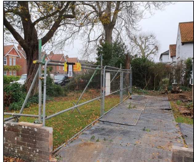
GP2: Tree protection barriers & trackmat ground protection
