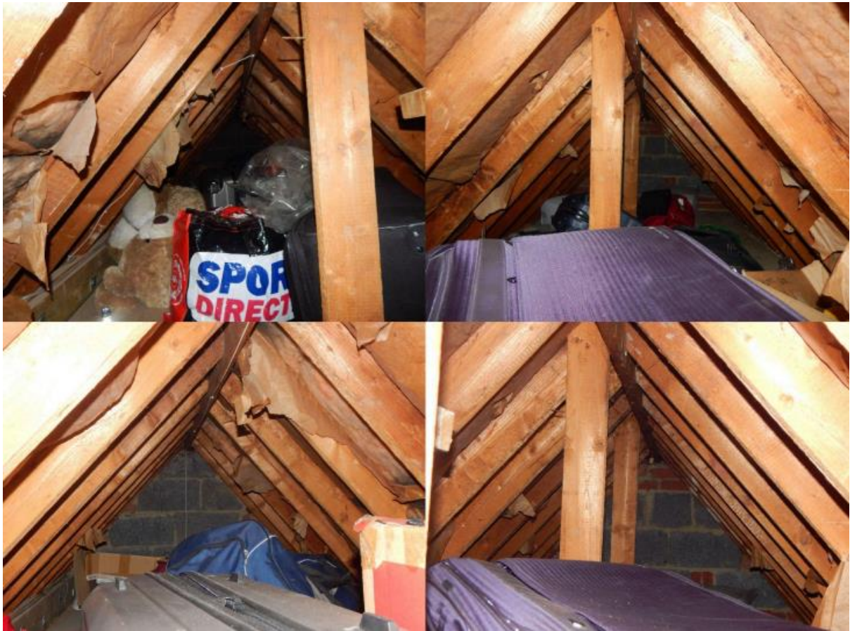
Image 7 – Internal views from within the main roof void spaces
