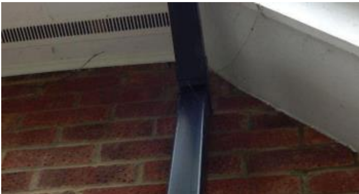
Image 6 – Close view of the eaves coverings to show condition throughout
