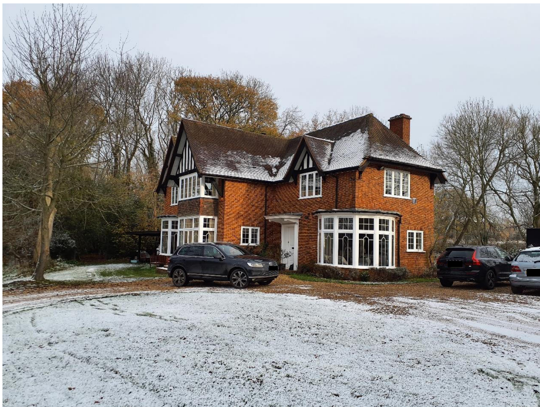
Figure 2 – Front of the property looking from south-west.
