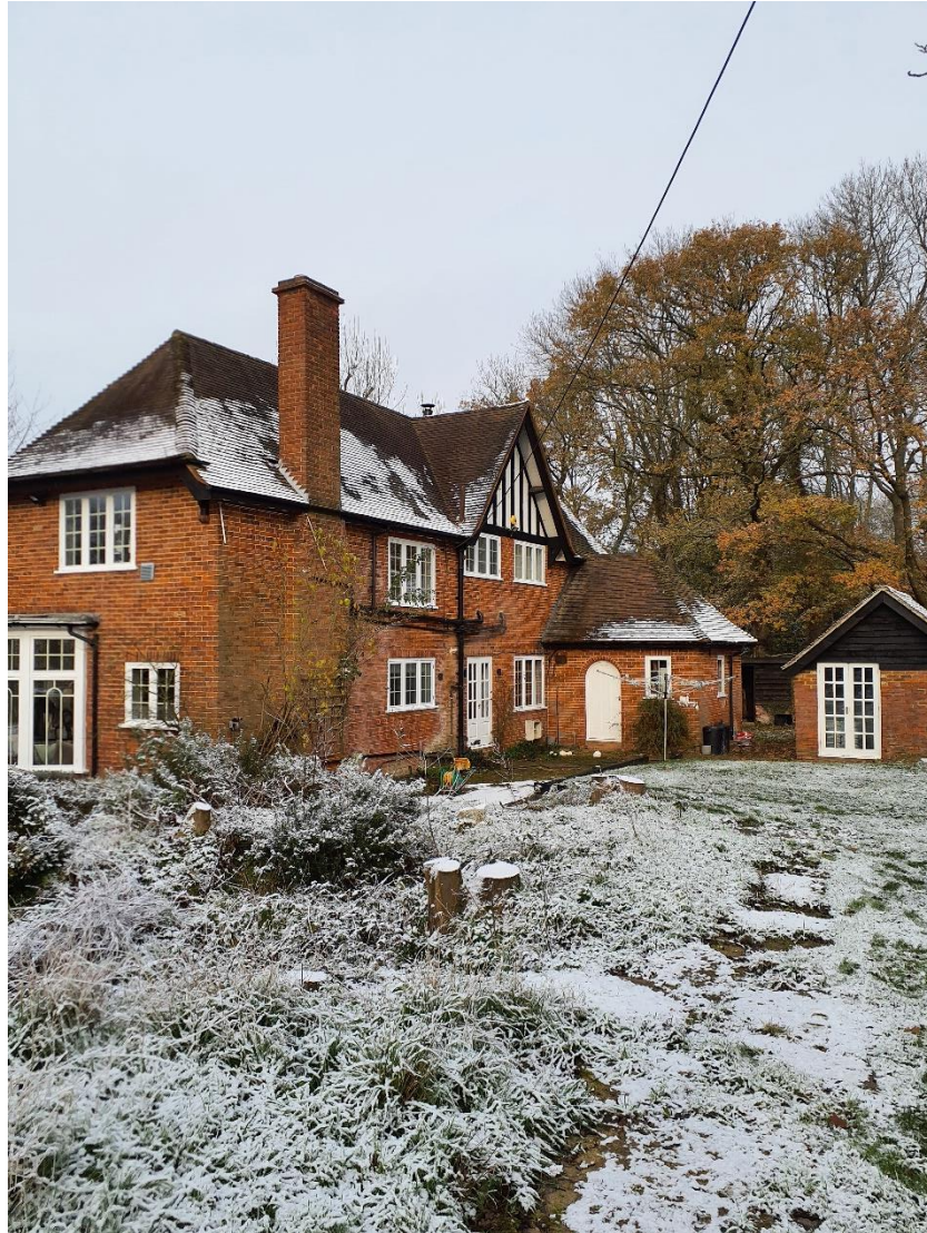
Figure 1 – Rear of the property looking towards the proposed extension site.
