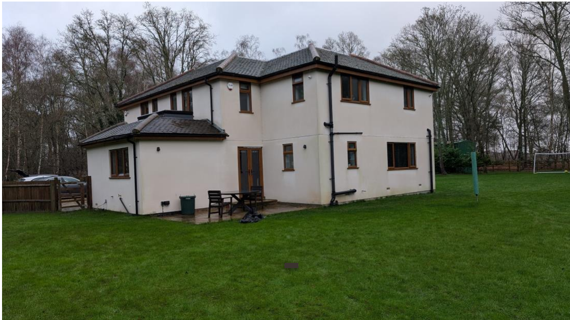
Image 03: Photograph of the existing side elevation.
