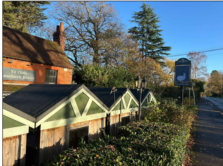
Rear image of existing huts
