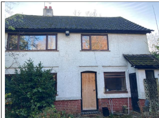
Photo 1 South west elevation
