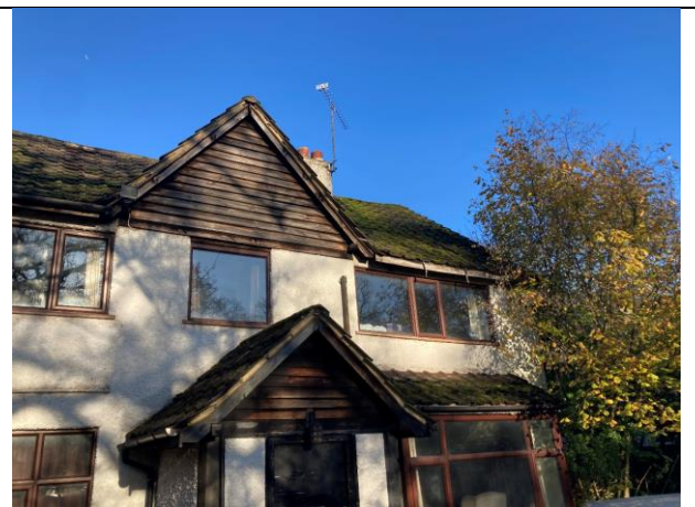
Photo 2 North east elevation
