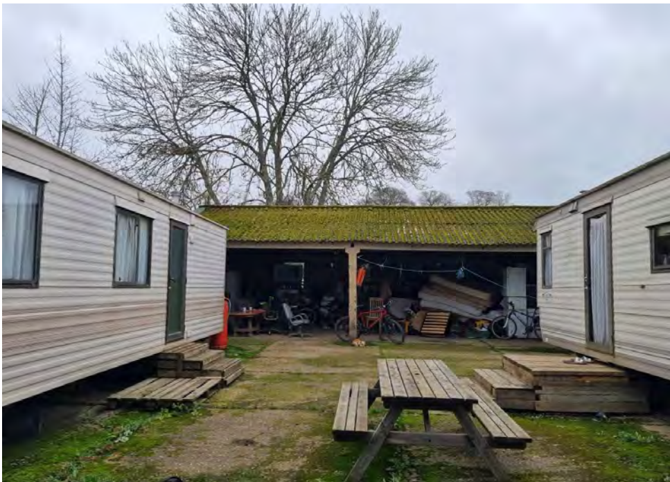
Photograph 6: Two caravans and open-sided barn situated in the centre/east of the Site (facing northeast).
