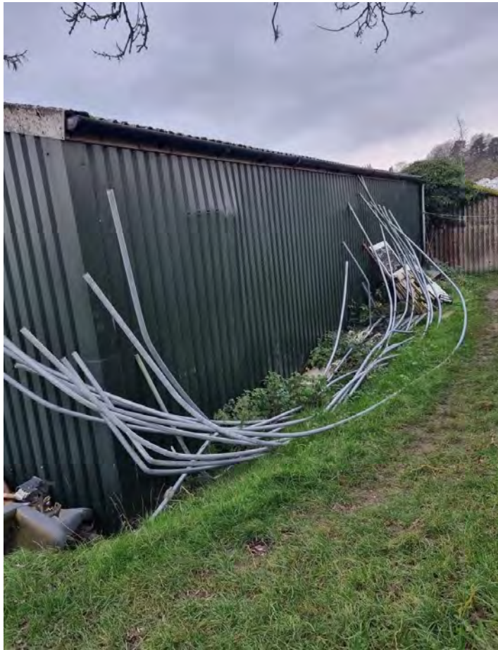
Photograph 7: Exterior view of one of the existing barns, including miscellaneous agricultural / waste material. Potential ACMs are present within the barn's building fabric.
