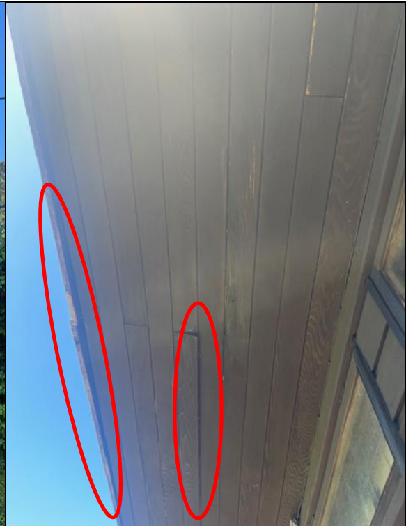
Photograph 2: Small gaps in exterior cladding. Summer house.
