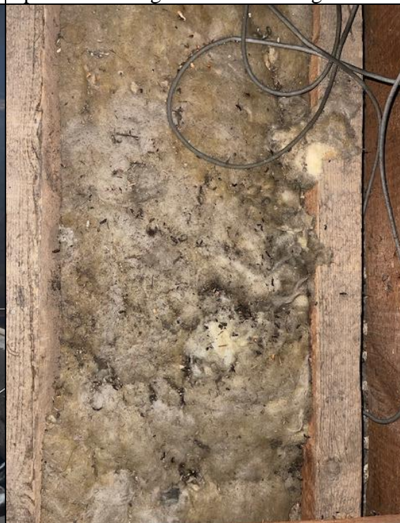
Photograph 16: Concentrated bat droppings in loft space. GTO original front building.
