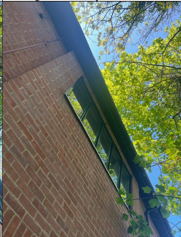
Photograph 8: Gaps in soffits. GTO House rear extension.
