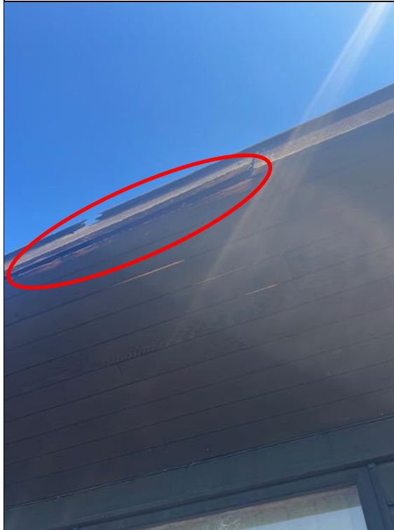
Photograph 3: Small gaps in exterior cladding. Summer house.
