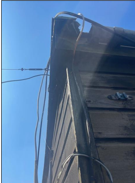
Photograph 5: Small gaps in exterior cladding. Summer house.
