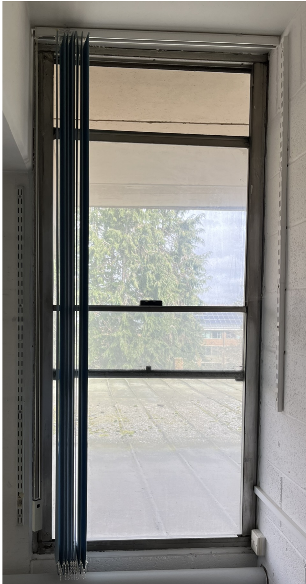
Existing sliding sash window (Level 3)
