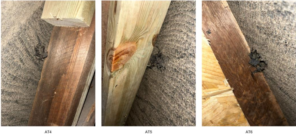
Figure 5 - Internal view showing holes through felt for Access Tiles 4-6
