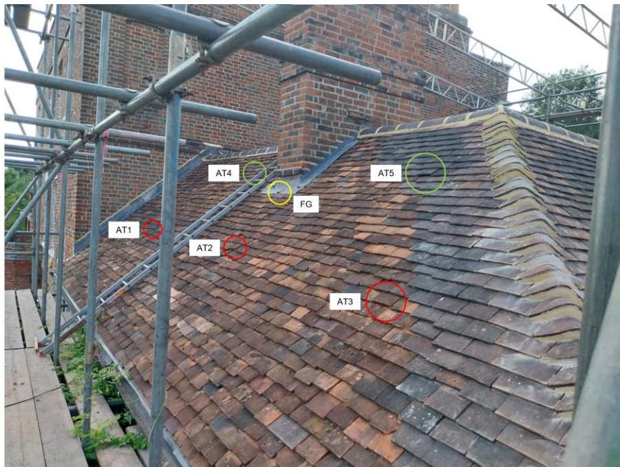
Figure 3 - Bat Access Provisions on Rear Flank
