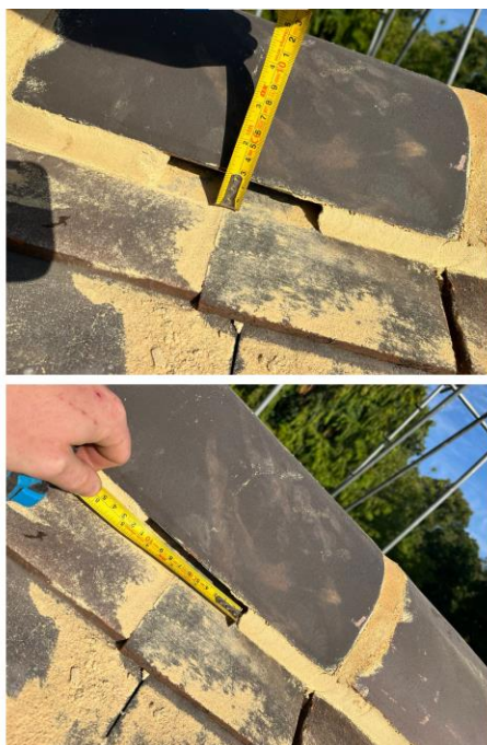
Figure 8 - Dimensions of Ridge Access Point
