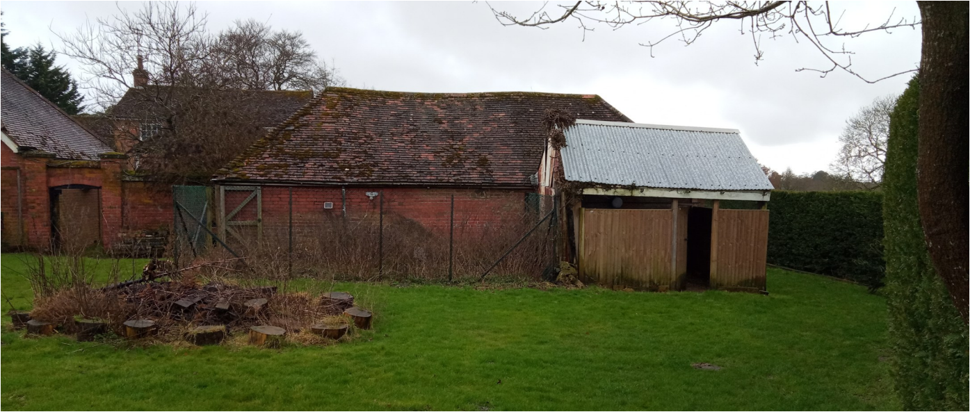
A) View of fenced chicken run and coop from north-east
