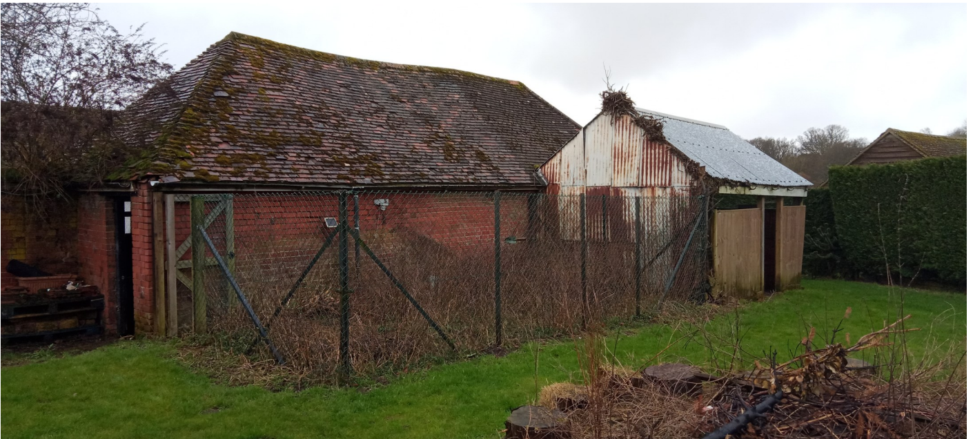
B) Chain link fencing forming chicken run with corrugated metal clad gable end and roof of chicken coop
