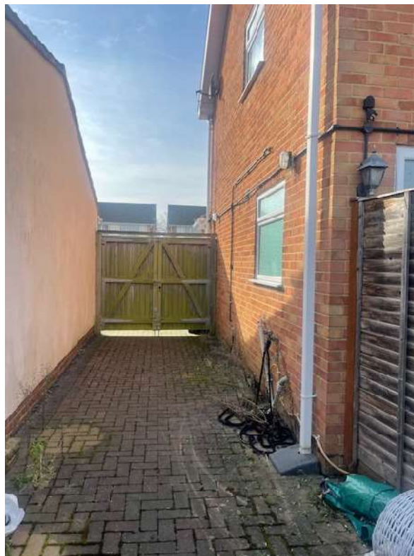
Figure 1. Existing Side Way
