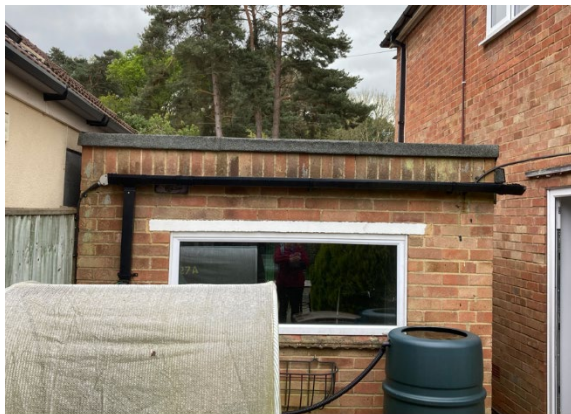
Photograph 9. Timber constructed roof with bitumen roofing felt (rear elevation)
