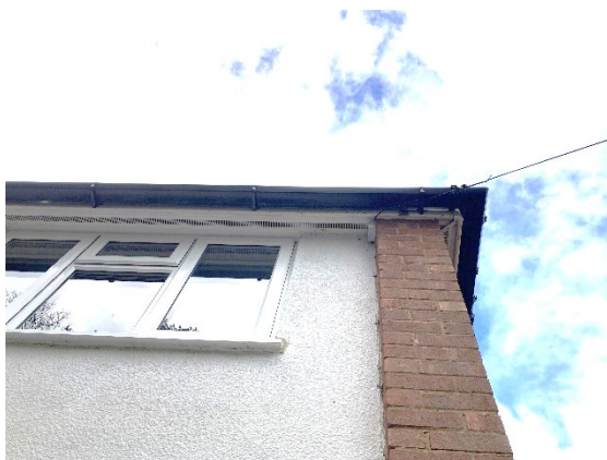
Photograph 7. Vented uPVC soffit tightly fit against the brickwork (front elevation).
