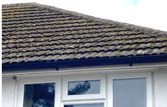
Photograph 4. Ridge and hip mortar fully intact (front elevation).
