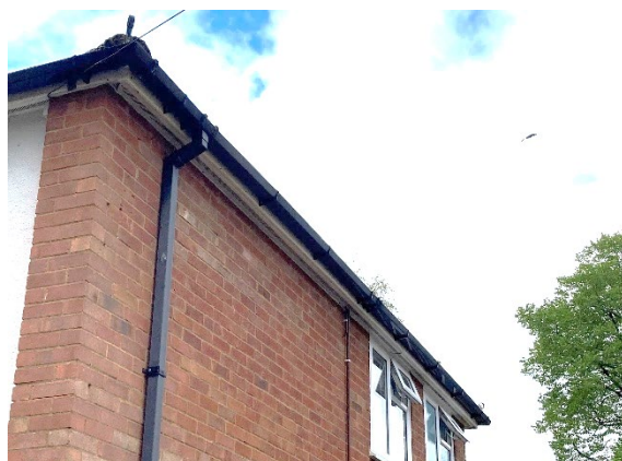
Photograph 8. uPVC soffit sealed to the brickwork wall (corner of eastern side and rear elevation).
