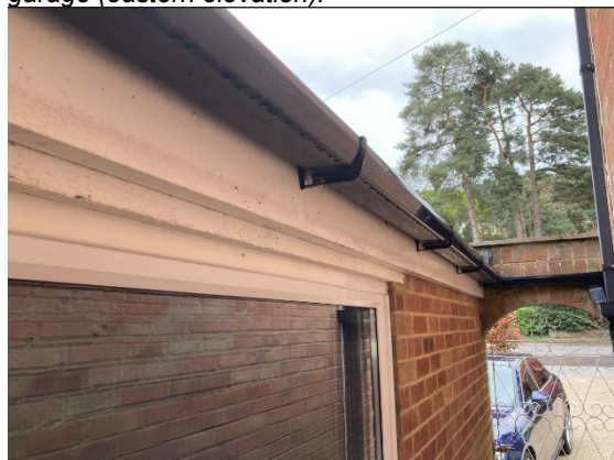
Photograph 12. Tightly fitted timber barge boards
