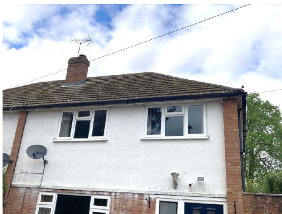
Photograph 1. Front elevation, viewed from the front.
