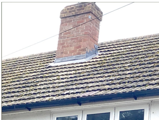
Photograph 3. Tight fitting interlocking concrete tiles (Front elevation)
