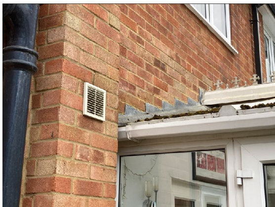
Photograph 5. Lead flashing sealed to the brickwork wall (rear elevation).
