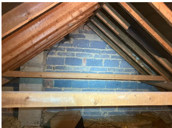
Photograph 13. Roof void showing 'cut and pitch' construction.
