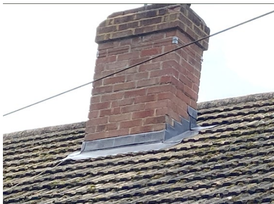
Photograph 6. Lead flashing well fitted but slightly raised around western chimney (front elevation).
