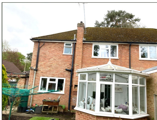
Photograph 2. Rear elevation, viewed from the rear.
