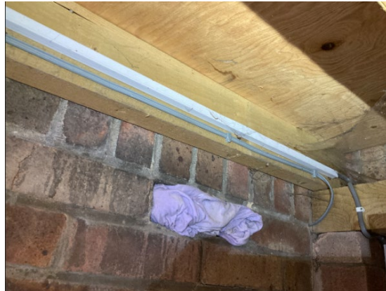
Photograph 10. Tightly fitted timber lining within the garage (eastern elevation).
