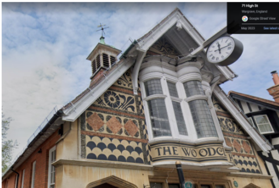
May 2023 (Google Street View) – Metal mesh guard to eaves and gable end of roof.
