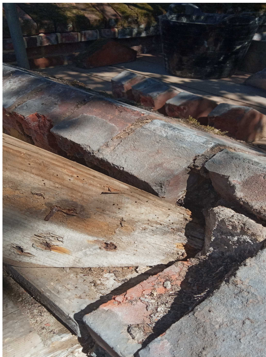
PHOTOS 1-3: Existing photos showing cut brick copings & rot to timbers
