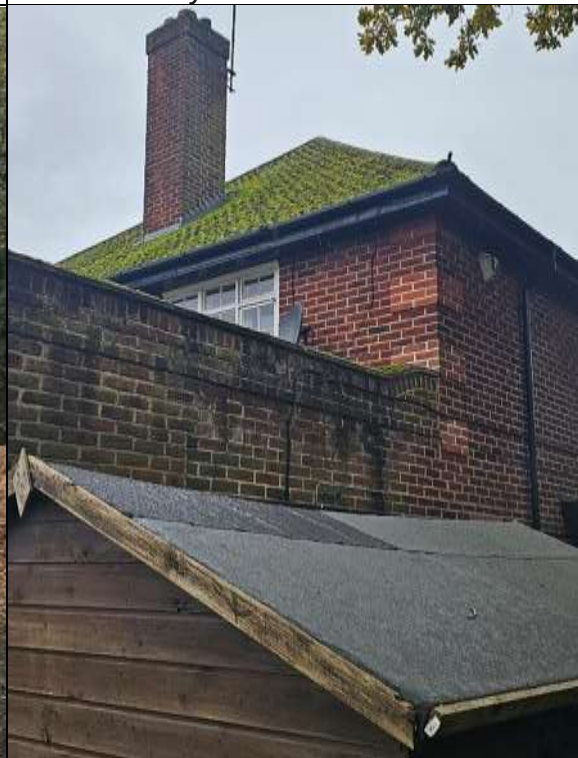
TN 4: Interlocking roof tiles in good condition no lifting or gaps.
