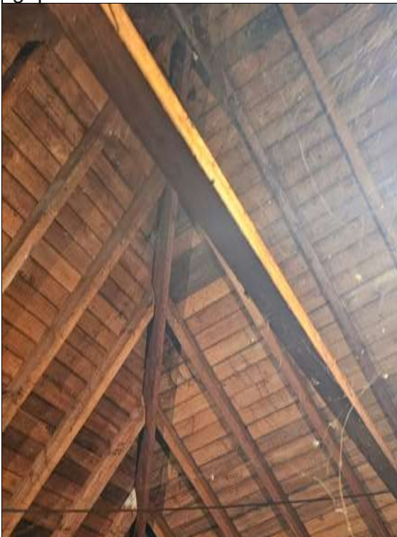
TN 7: Timber clad roof liner
