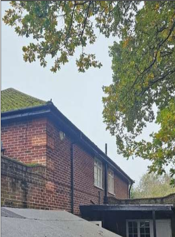
TN 5: Well-fitted tight soffits without gaps.
