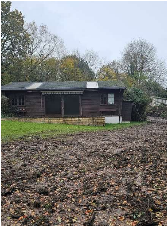
TN 1: Timber clad shed.
