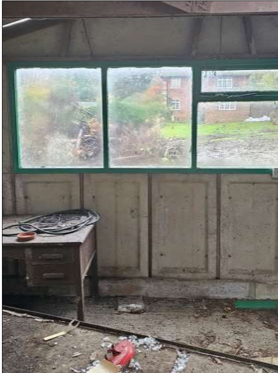
TN 13: Wooden outbuilding interior.
