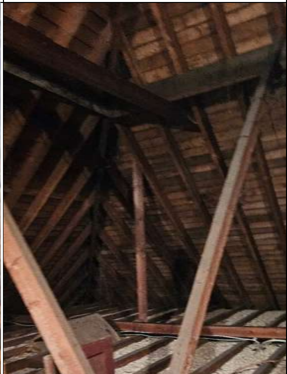
TN 8: Loft space of house.
