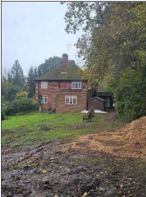
TN 3: Rear elevation of house.
