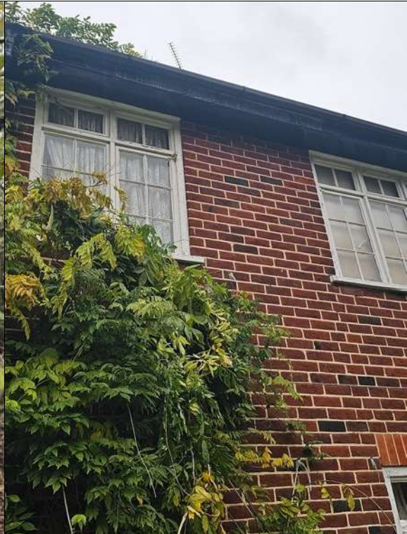
TN 18: Main house.
