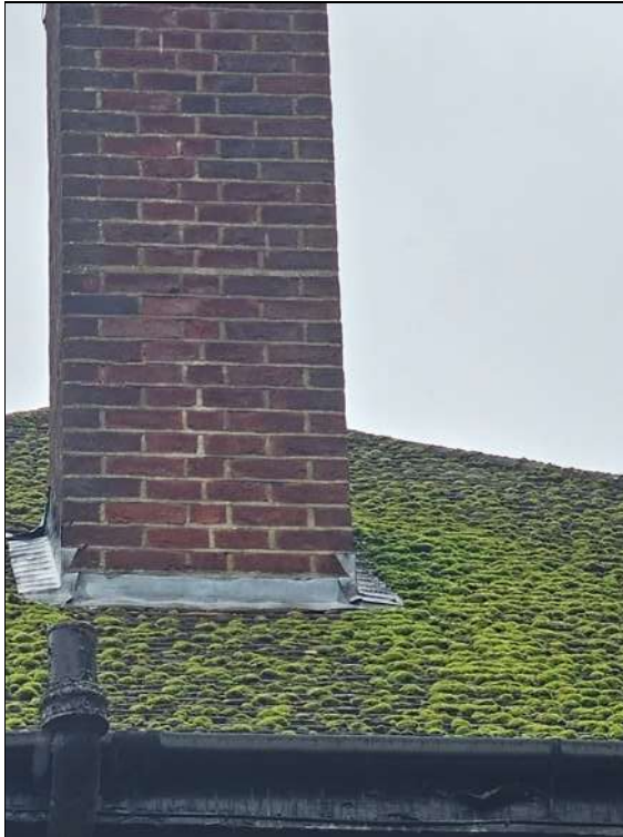
TN 9: Tight fitted lead flashing.
