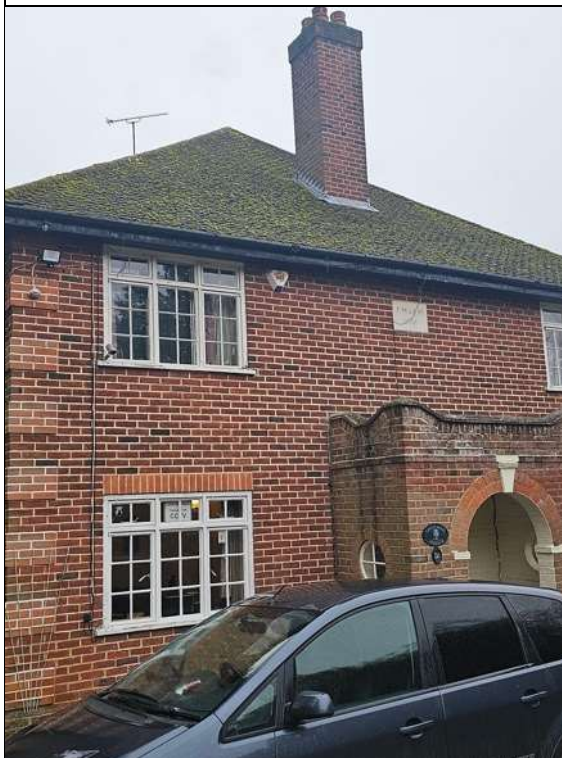
TN 19: Main house with no gaps in the roof tiles.
