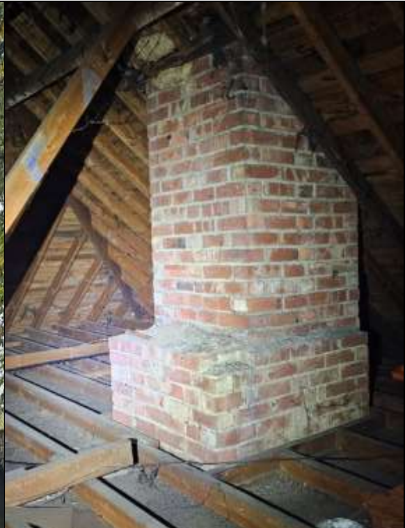
TN 6: Loft fully inspected.
