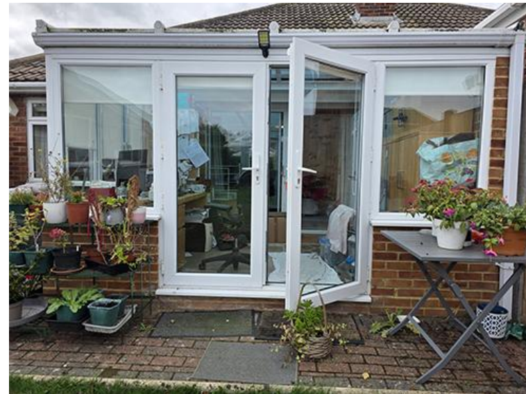
Existing rear conservatory
