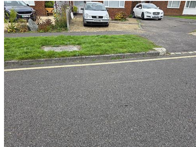
View of existing BT cover
