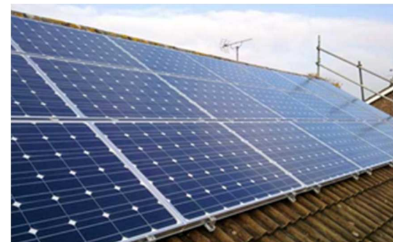
Picture 1 —Roof mounted PV panels
