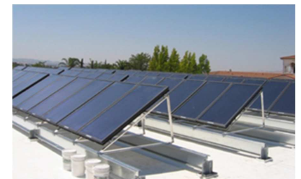
Picture 2—Frame mounted PV on flat roof
