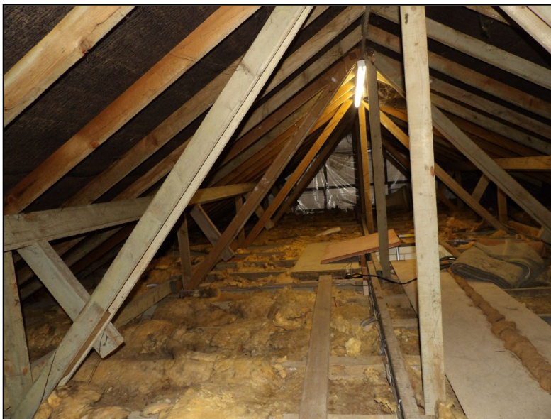
Figure 11. Example loft space/bitumen lining to tiles. 76 Arthur Road, Wokingham. 22.10.24
