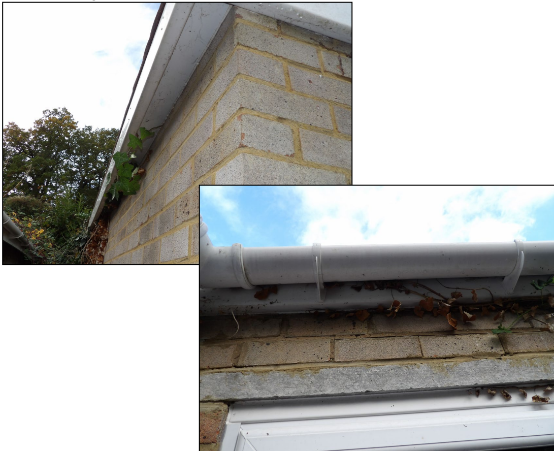
Figure 10. Tightly fitted soffits/fascias on garage/front porch/living space. 76 Arthur Road, Wokingham. 22.10.24
