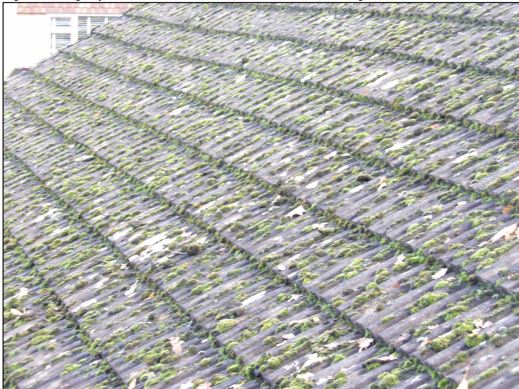
Figure 4. Tightly fitted roof tiles. 76 Arthur Road, Wokingham. 22.10.24
