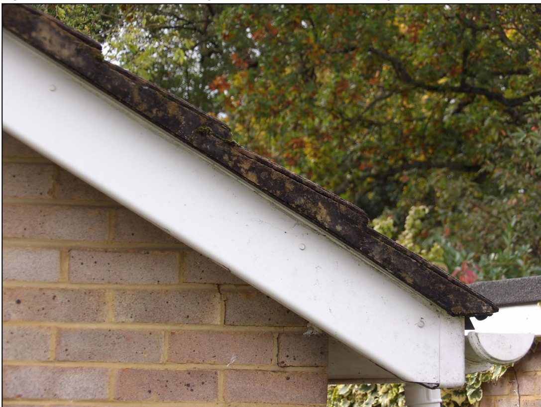
Figure 6. Example of sealed verges. 76 Arthur Road, Wokingham. 22.10.24
