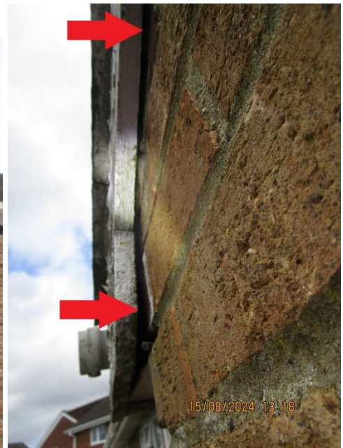
Photo 7 – Hole in the soffit box, and Photo 8 - Gap between the under cloaking and barge board on the front elevation
