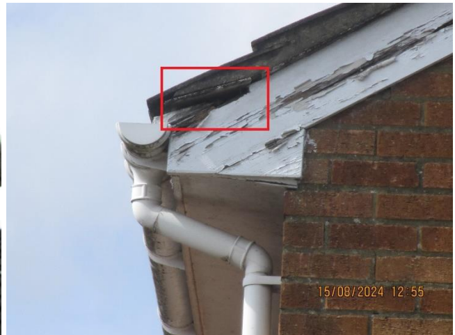
Photo 7 – Hole in the soffit box, and Photo 8 - Gap between the under cloaking and barge board on the front elevation
