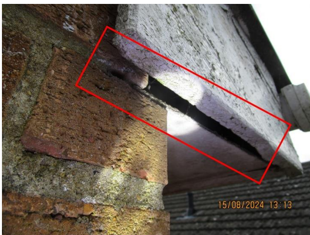
Photo 7 – Hole in the soffit box, and Photo 8 - Gap between the under cloaking and barge board on the front elevation
