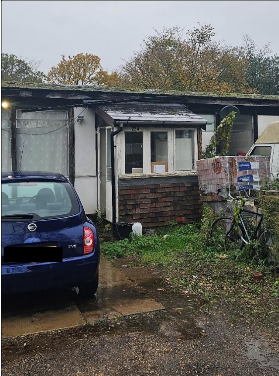
Photograph 3: Front elevation – no gaps around roof tiles.
