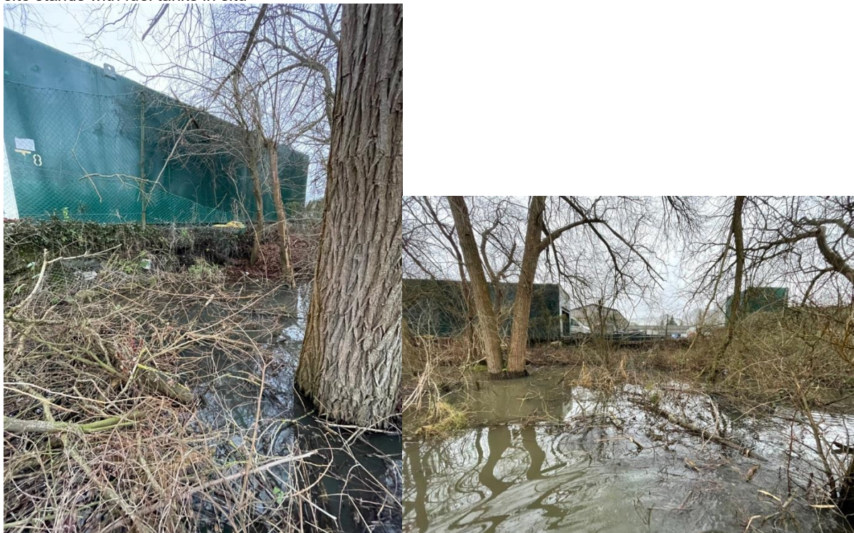
Photograph illustrating subsiding flood water up to site boundary and the unretained made ground on which the site stands with fuel tanks in situ
