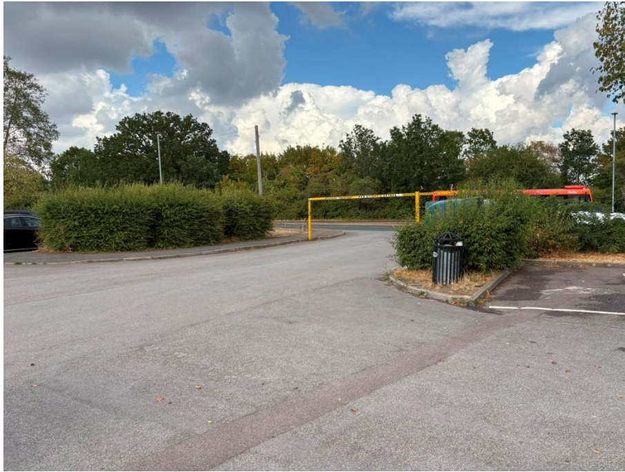
Image 3 – Entrance car park to the north of the site
