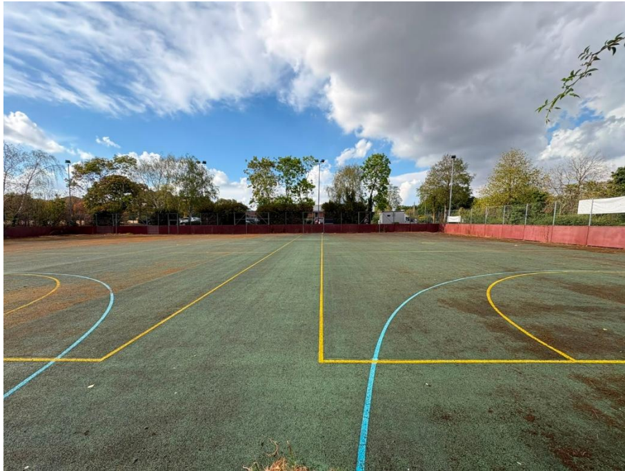
Image 1 – Existing porous asphalt netball courts
