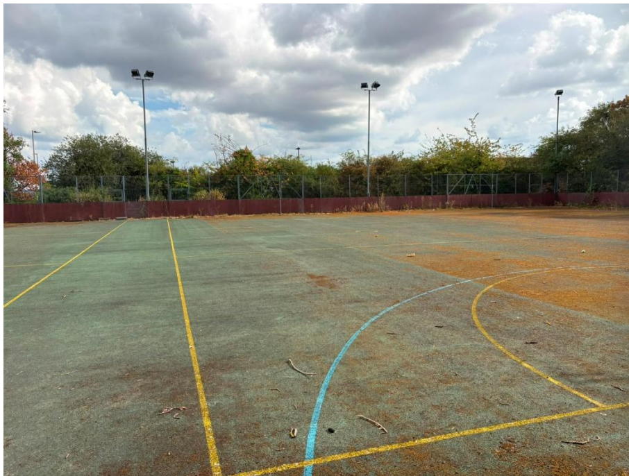
Image 2 – Existing porous asphalt netball courts
