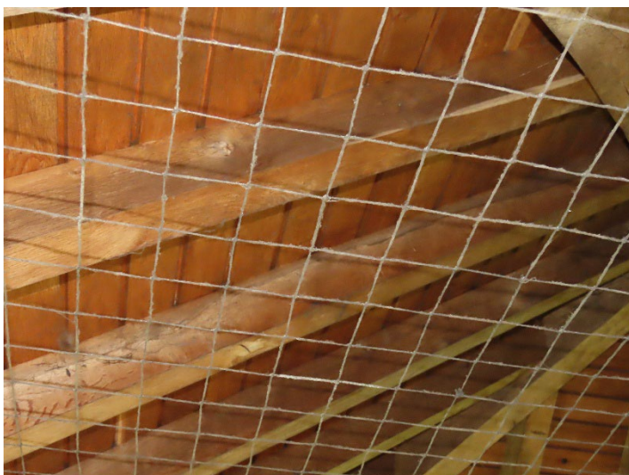
Plate 3. General view of internal side of roof
