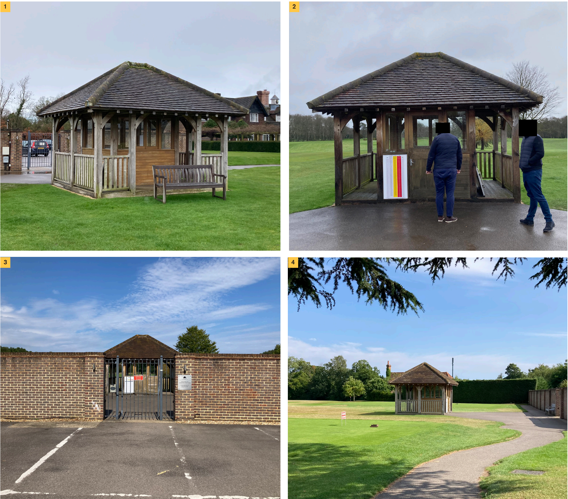
Figure 4. Photographs of Existing Starters Hut
