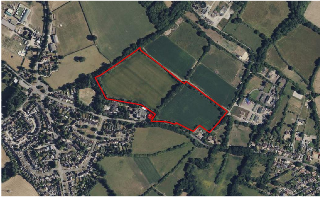
Figure 1: Site location shown on Google aerial image
