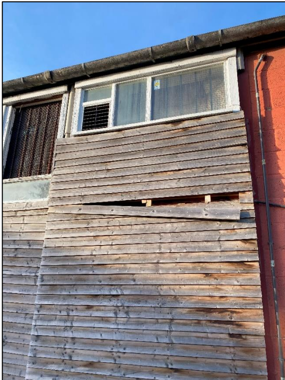
Image 2: Slipped wooden boards on B2
