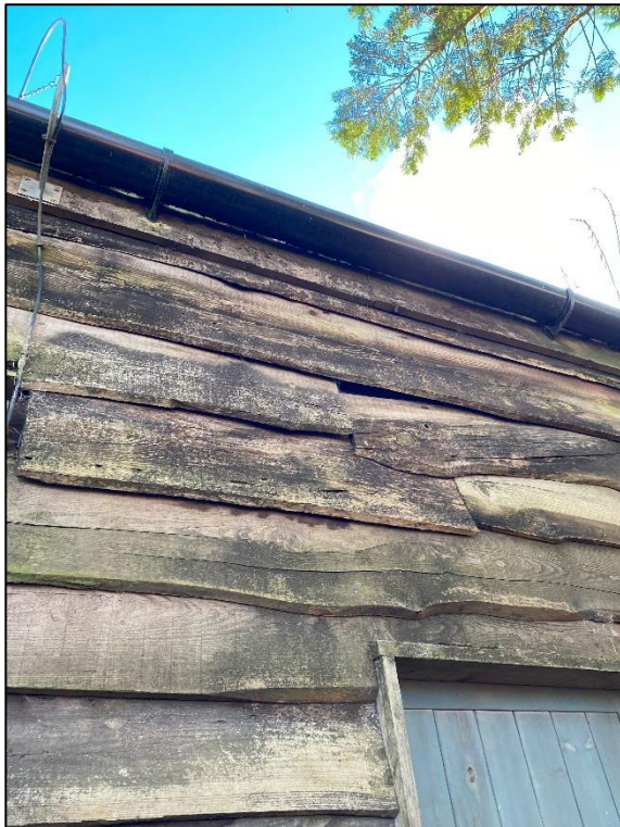
Image 4: Example of slipped wooden cladding on B5
