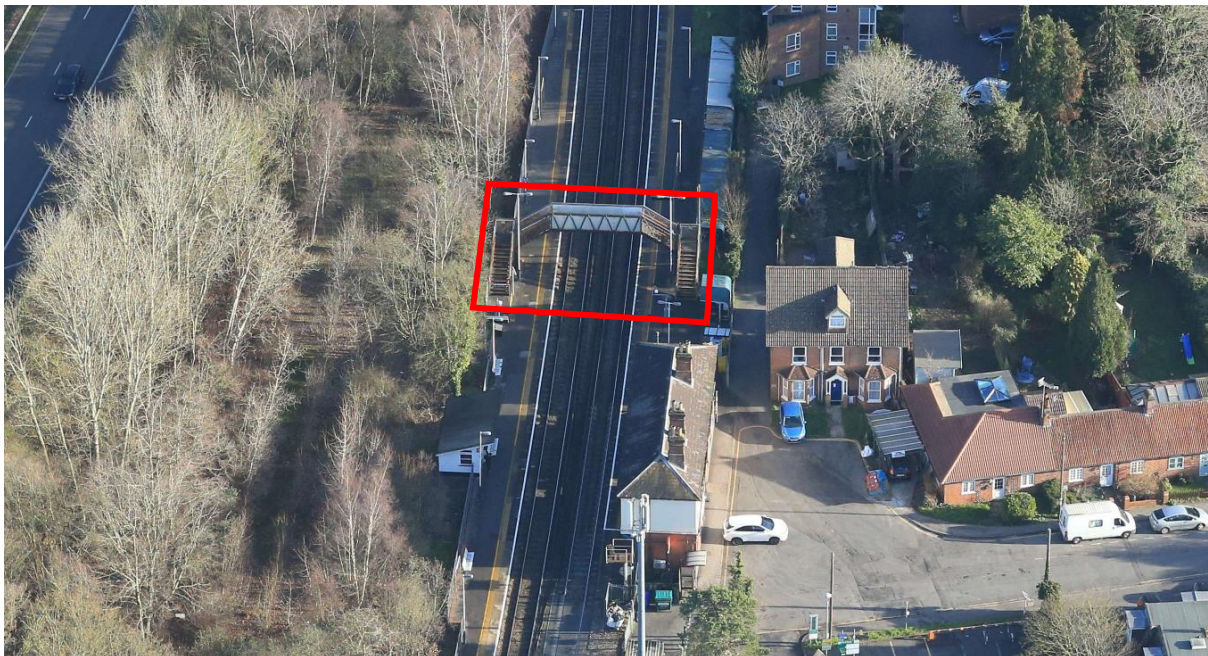
Figure 3 – Aerial photograph of Earley Station Footbridge looking east (January 2019).
