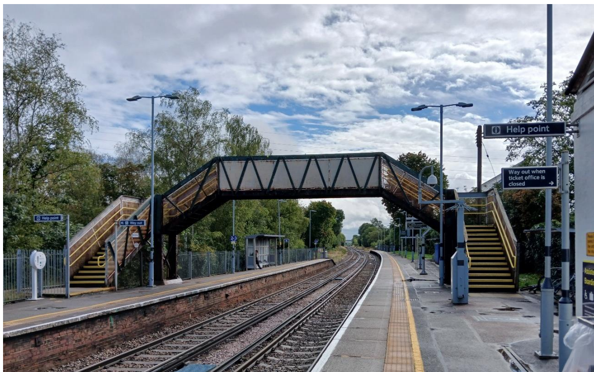
Figure 1 - Photograph of Earley Footbridge
