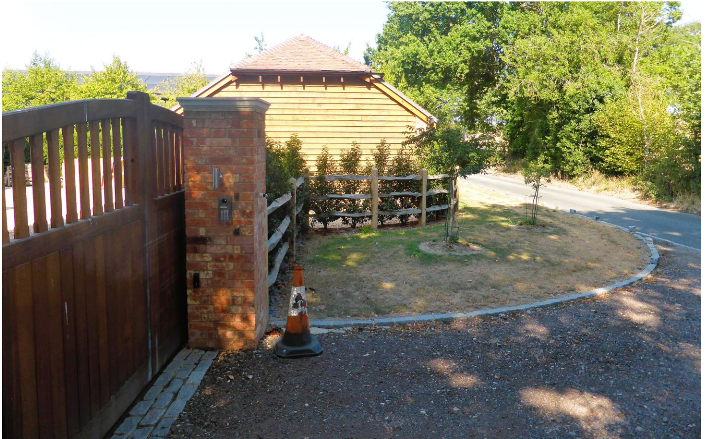
PHOTO 1. Front gate and piers on the left. New planting and timber fence centre, amended cladding on end elevation of approved building.
