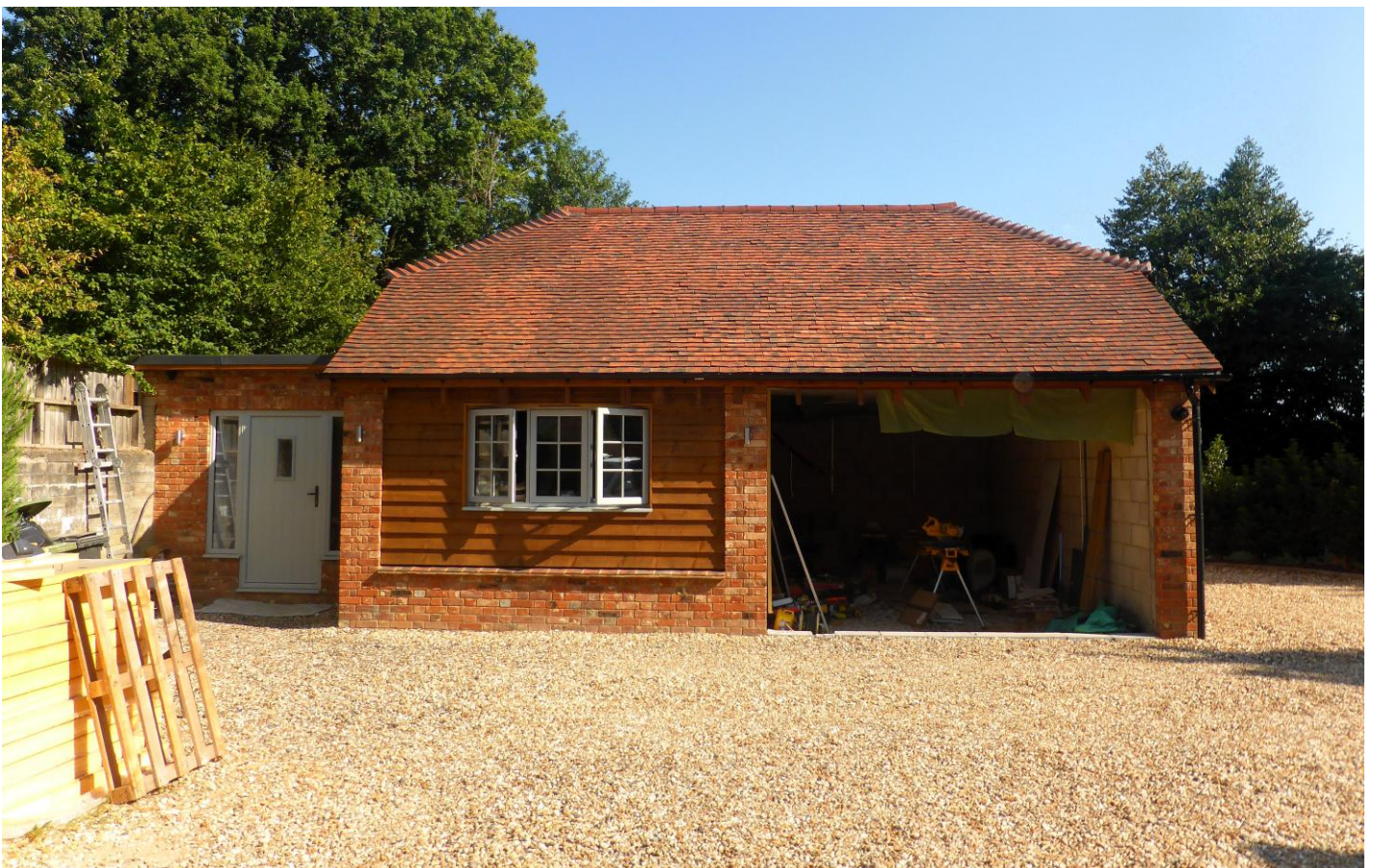
PHOTO 2. Amended principal elevation showing enclosure of garage, addition of window and change to door surround by addition of glazing.
