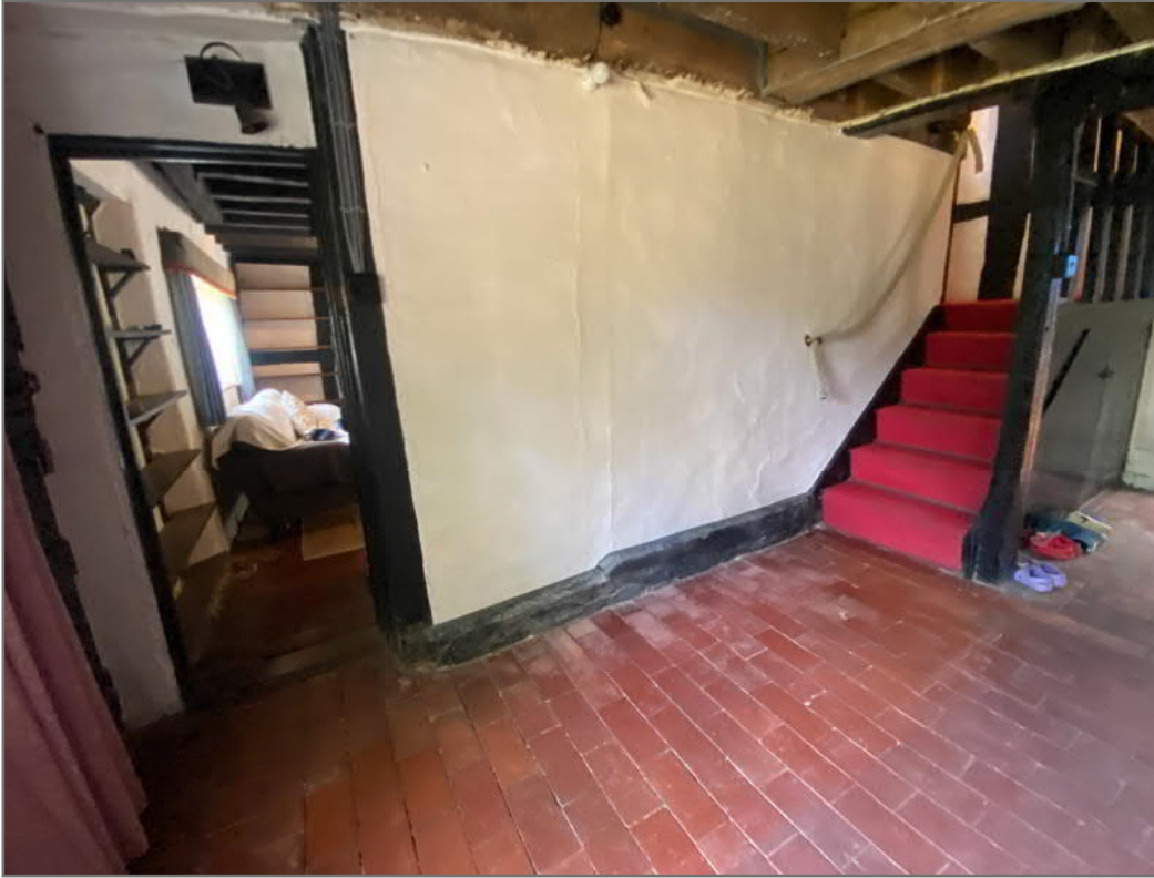
Image 9: View of staircase, and through doorway to Lounge beyond
