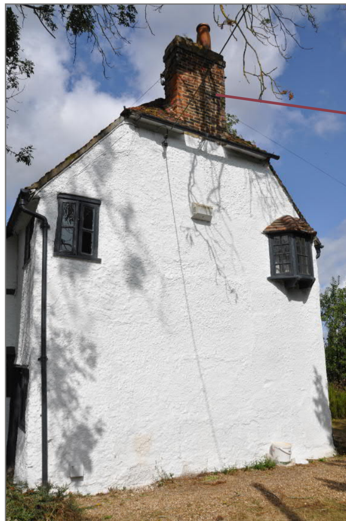
Image 3: South elevation (Phase 1 construction)
