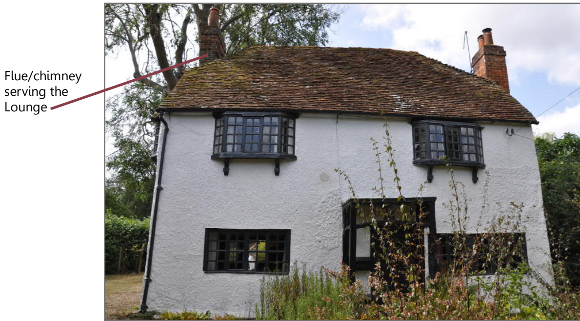
Image 2: East elevation (Phase 1 construction)
