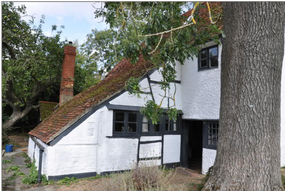
Image 4: South elevation of outshut and catslide roof (Phase 2 construction)
