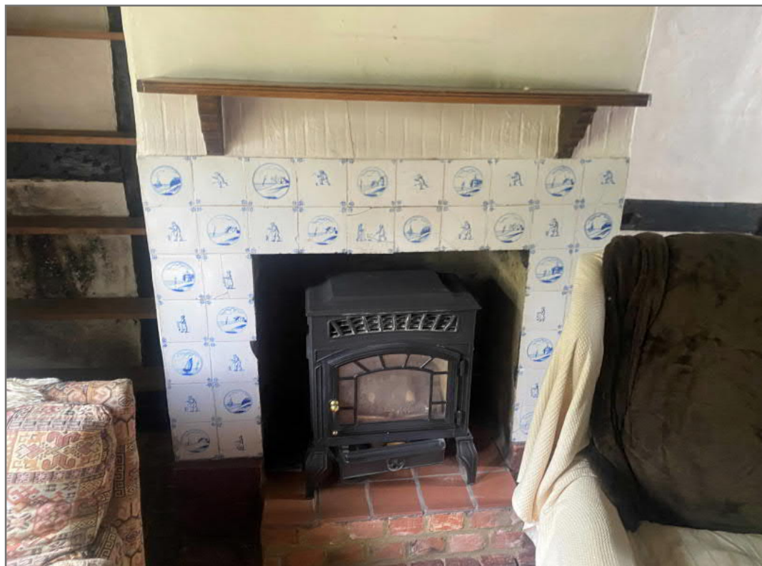
Image 8: View of previous gas stove removed in August 2024 after found unsafe
