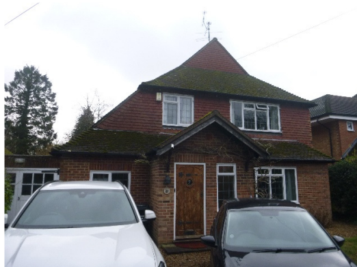
Photograph 1. Front of the detached dwelling viewed from the west.
