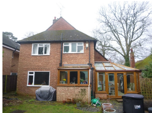
Photograph 2. Rear of the detached dwelling viewed from the east.
