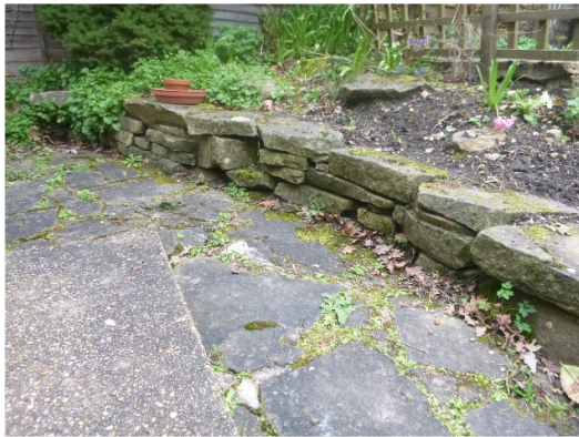
Photograph 15. Stone wall on the edge of the patio to the rear eastern side of the house.
