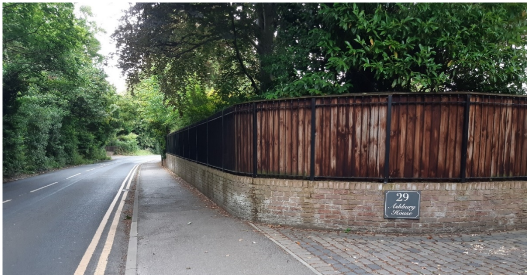
Fig. 1: External boundary treatment at no. 29 Wiltshire Road, Wokingham
