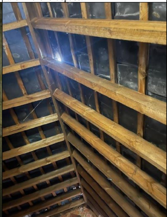
Photograph 12: Loft space, light coming through at ridge.
