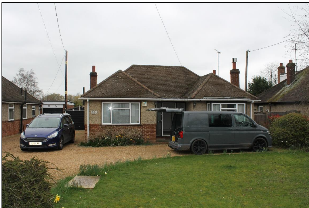
Photograph 1 – Front elevation as viewed from Danywern Drive
