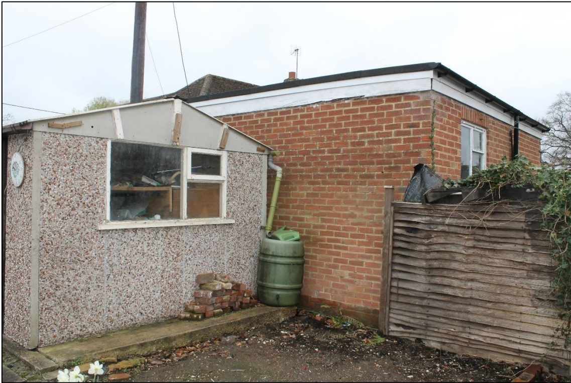
Photograph 4 – Detached garages to No. 10 and No. 8 Danywern Drive as viewed from the rear garden to No. 10 Danywern Drive
