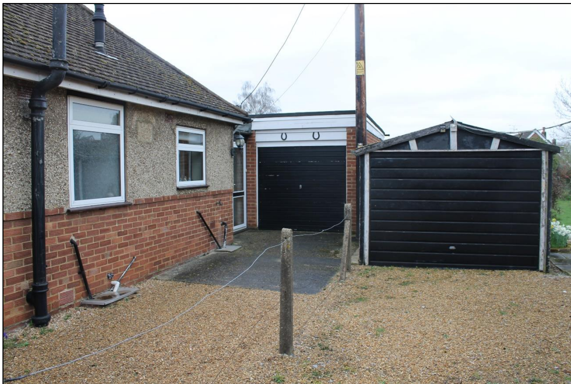
Photograph 1 – Windows to side elevation of No. 8, Danywern Drive
