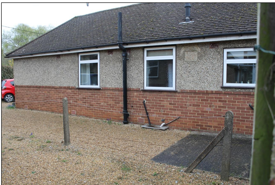
Photograph 2 – Windows to side elevation of No. 8, Danywern Drive (Window 1 on the right-hand side and window 2 on the far left-hand side)
