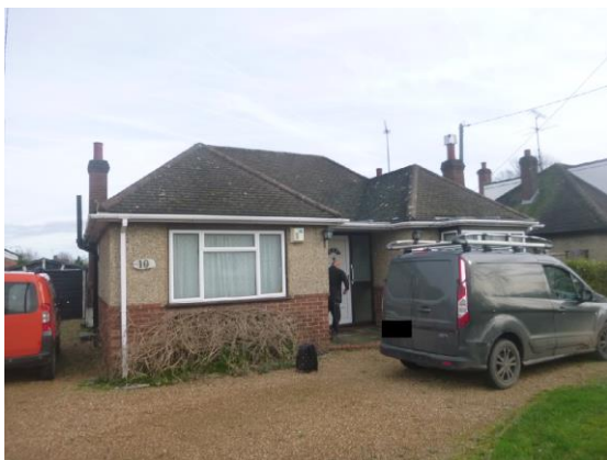
Photograph 1. Front of property viewed from southwest.
