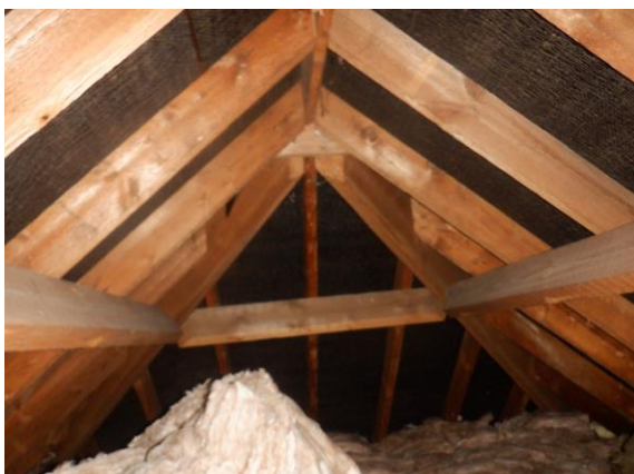
Photograph 11. Fully intact bitumen felt roof lining.
