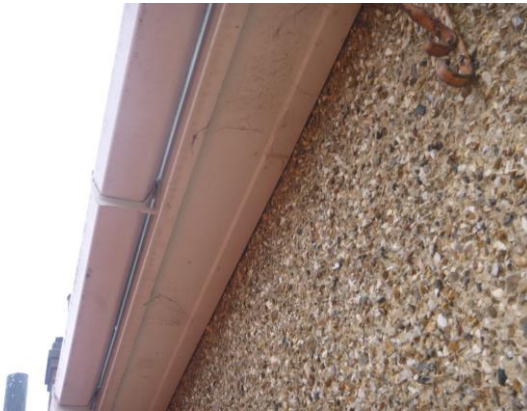
Photograph 8. uPVC soffit sealed to the rendered wall (northwest elevation).
