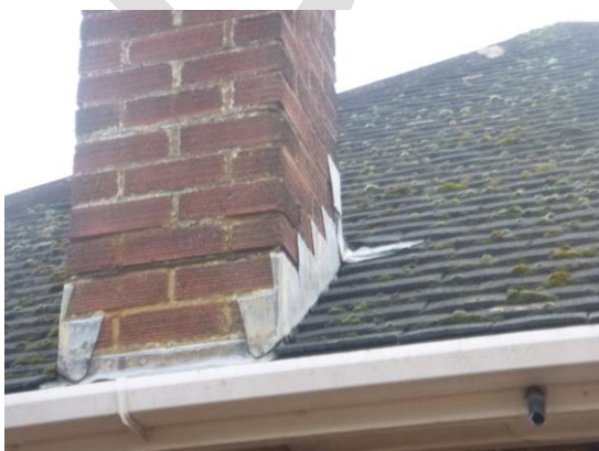
Photograph 5. Lead flashing sealed to brickwork and roof tiles (northwest elevation).
