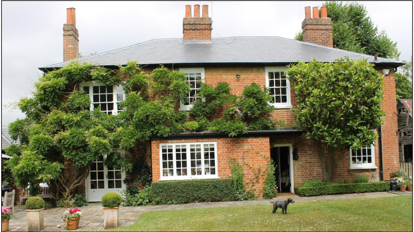
Photograph 3 – Rear elevation showing the single-storey extension to the original dwelling
