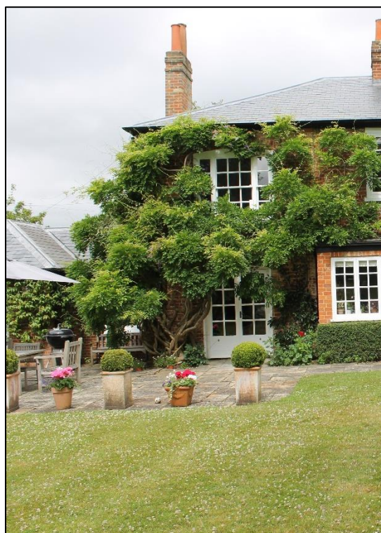
Photograph 2 – Rear elevation showing the two-storey side extension to the original dwelling
