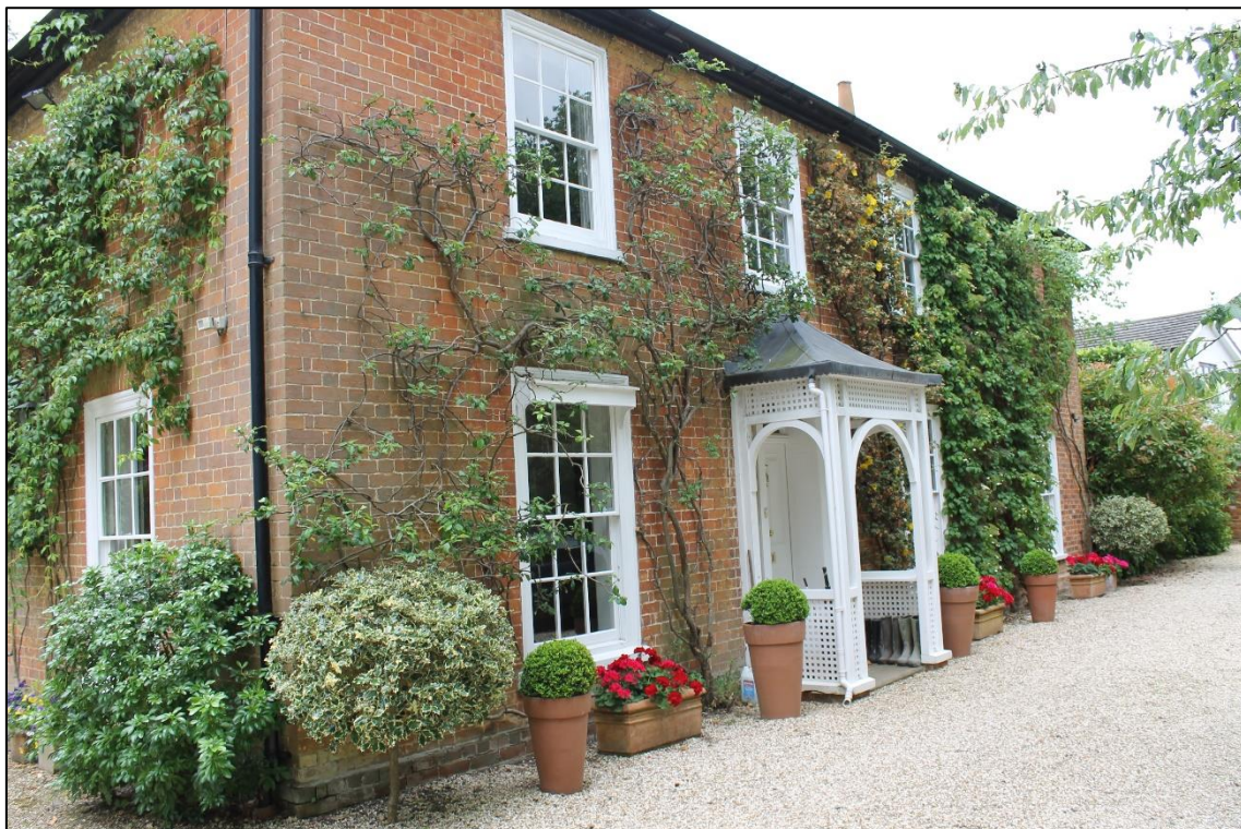
Photograph 1- Front elevation as viewed from the driveway
