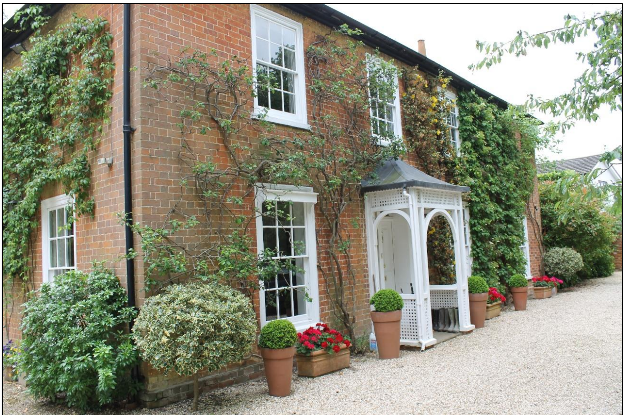
Photograph 1- Front elevation as viewed from the driveway
