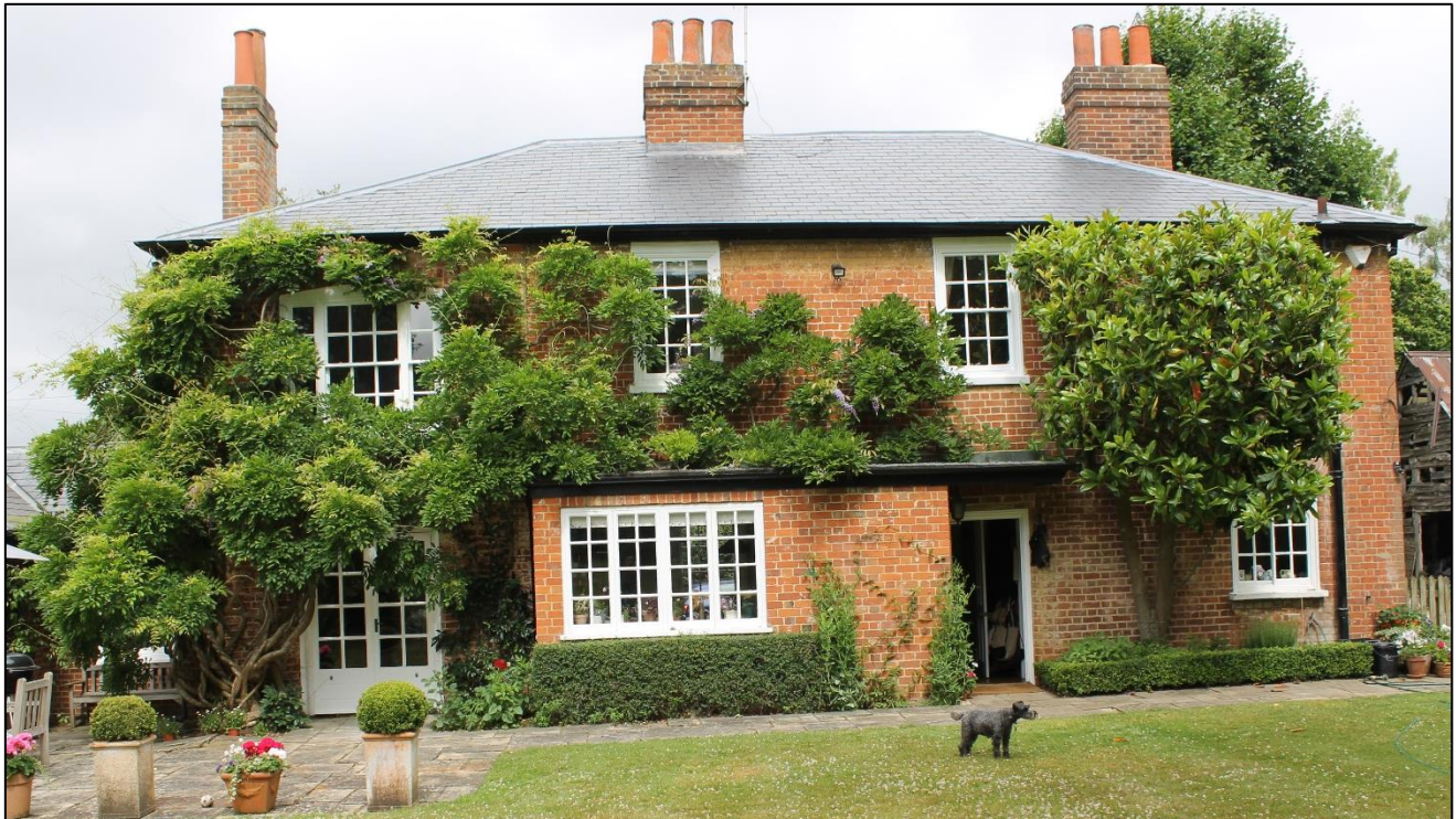
Photograph 2 – Rear elevation as viewed from the garden
