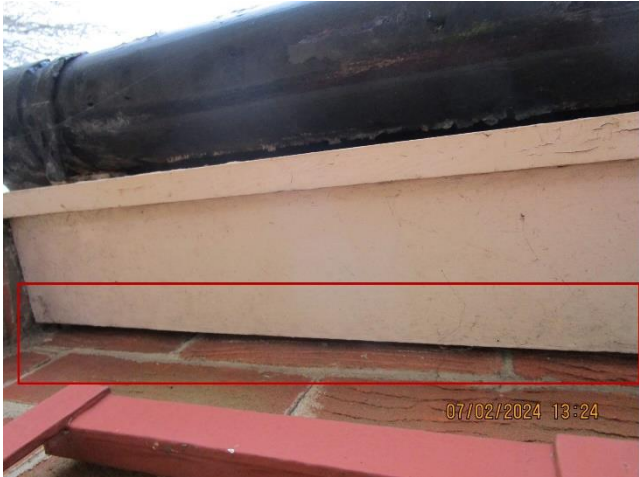
Photos 17 and 18 – Gaps under tiles above the walls where the roof has sagged in relation to the walls (garage)
