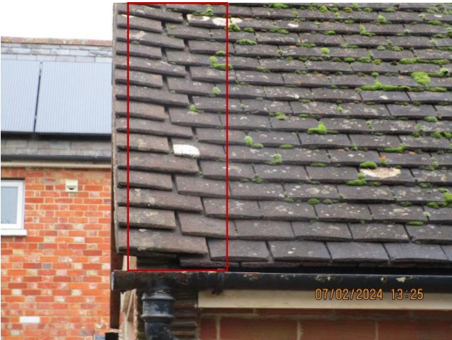
Photos 17 and 18 – Gaps under tiles above the walls where the roof has sagged in relation to the walls (garage)
