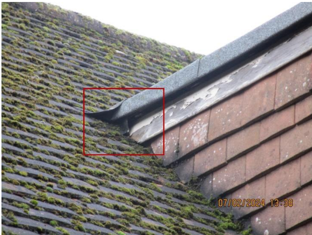
Photo 7 – Gap at the intersection of the roofs, and, Photo 8 – Gap where the dormer window meets the main roof
