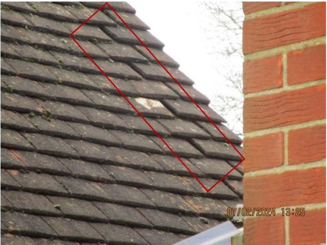
Photos 17 and 18 – Gaps under tiles above the walls where the roof has sagged in relation to the walls (garage)
