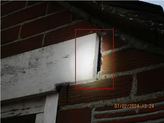
Photos 17 and 18 – Gaps under tiles above the walls where the roof has sagged in relation to the walls (garage)
