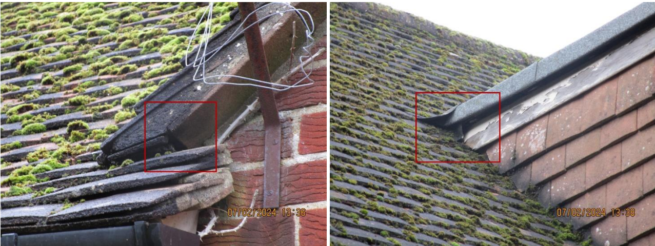
Photos 9 and 10 – Inside the two loft spaces
