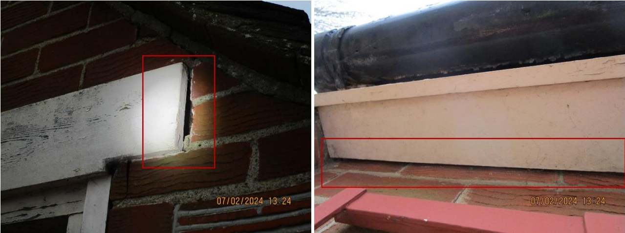
Photos 17 and 18 – Gaps under tiles above the walls where the roof has sagged in relation to the walls (garage)
